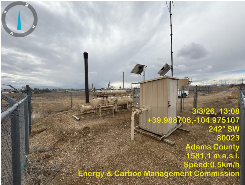
Photo 7 Separator, Gas Meter Run.
