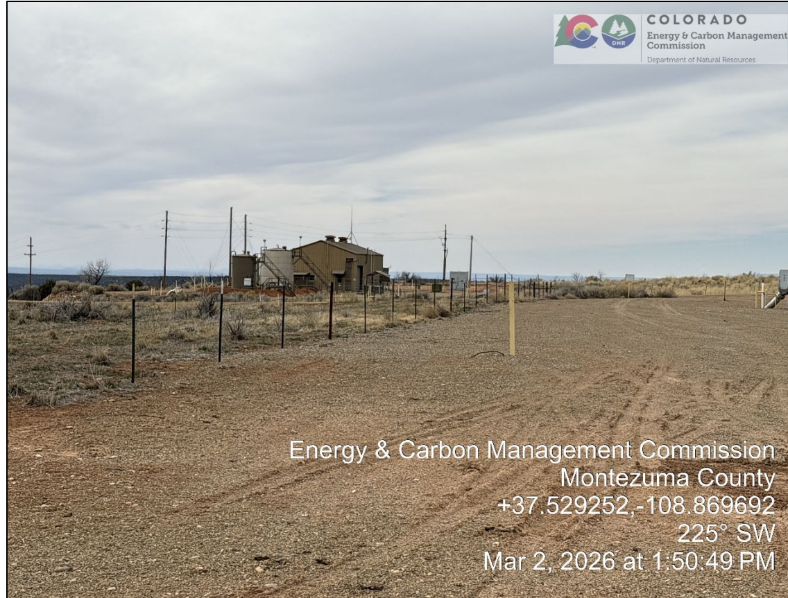
9. Pad margin and interim reclamation area separated by 4-strand barbed wire fence. Rig anchor marker.
