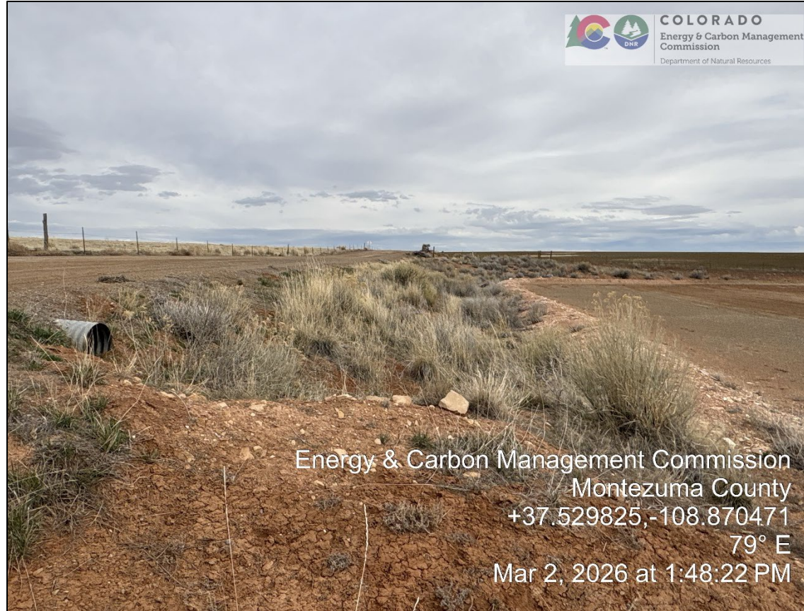
6. Stormwater ditch and berm fed by culvert from county road.
