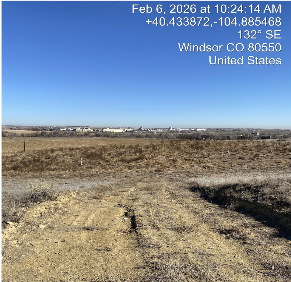
Photo 1. Photo taken from access road looking down on location. Access road has not been reclaimed and remains bare. Due to this there is a high risk stormwater erosion.
