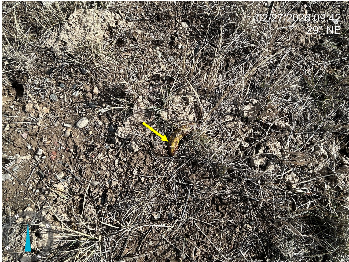
Photo 3: Photos showing an unmarked guy line anchor located in the southeastern interim area. Comply with Rule 1003.a. and mark or remove anchor.
