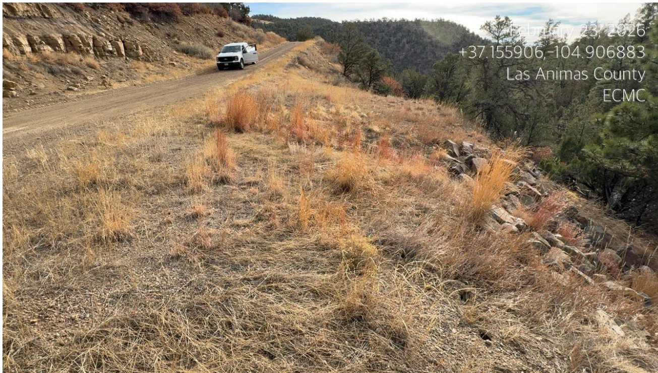
Photo 2. The former location is revegetated and stabilized. The location will need to be recontoured upon access road reclamation in the future.
