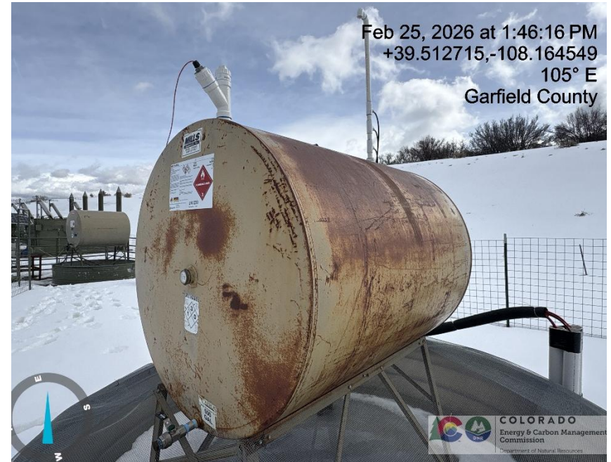
Photo # 4029 Methanol tank lacks operator contact info & 911, additionally tank labeled with previous operator name
