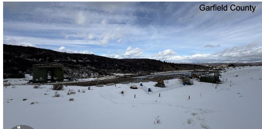
South West corner of location.
