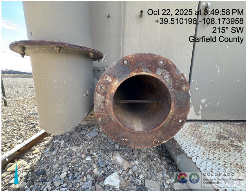
Photo # 1783 From inspection/audit 708907747 conducted on 10/22/2025 Fire tube open ended/wildlife hazard /available for entry by wildlife
