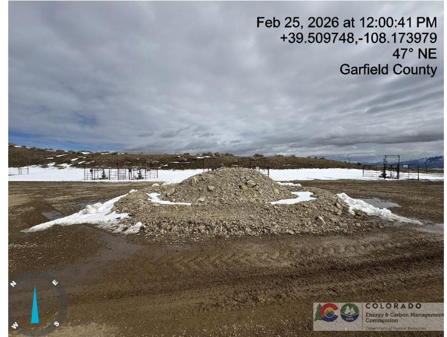
Photo # 3758 Soil & rock stockpile with berm
