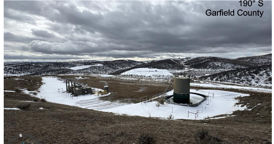
North East corner of location.
