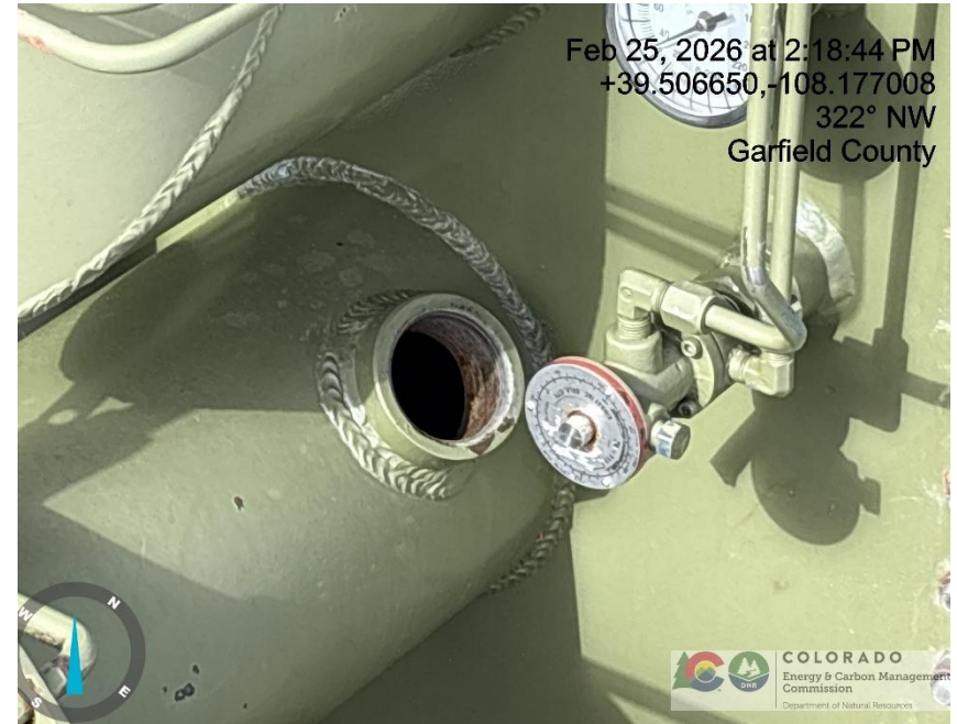
Photo # 4176 Open ended pipe on fire tube/wildlife hazard /available for entry by wildlife
