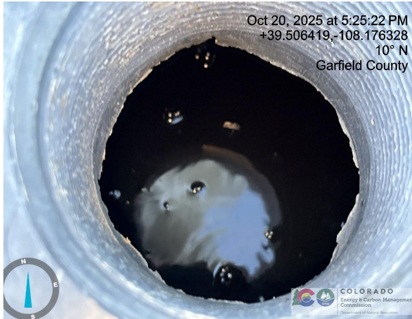
Photo # 687 From inspection/audit 708907686 conducted on 10/20/2025 - Failure to maintain chemical BMP – Chemical tank containment approximately 3/4 full of fluid/BMP insufficient to contain possible spill
