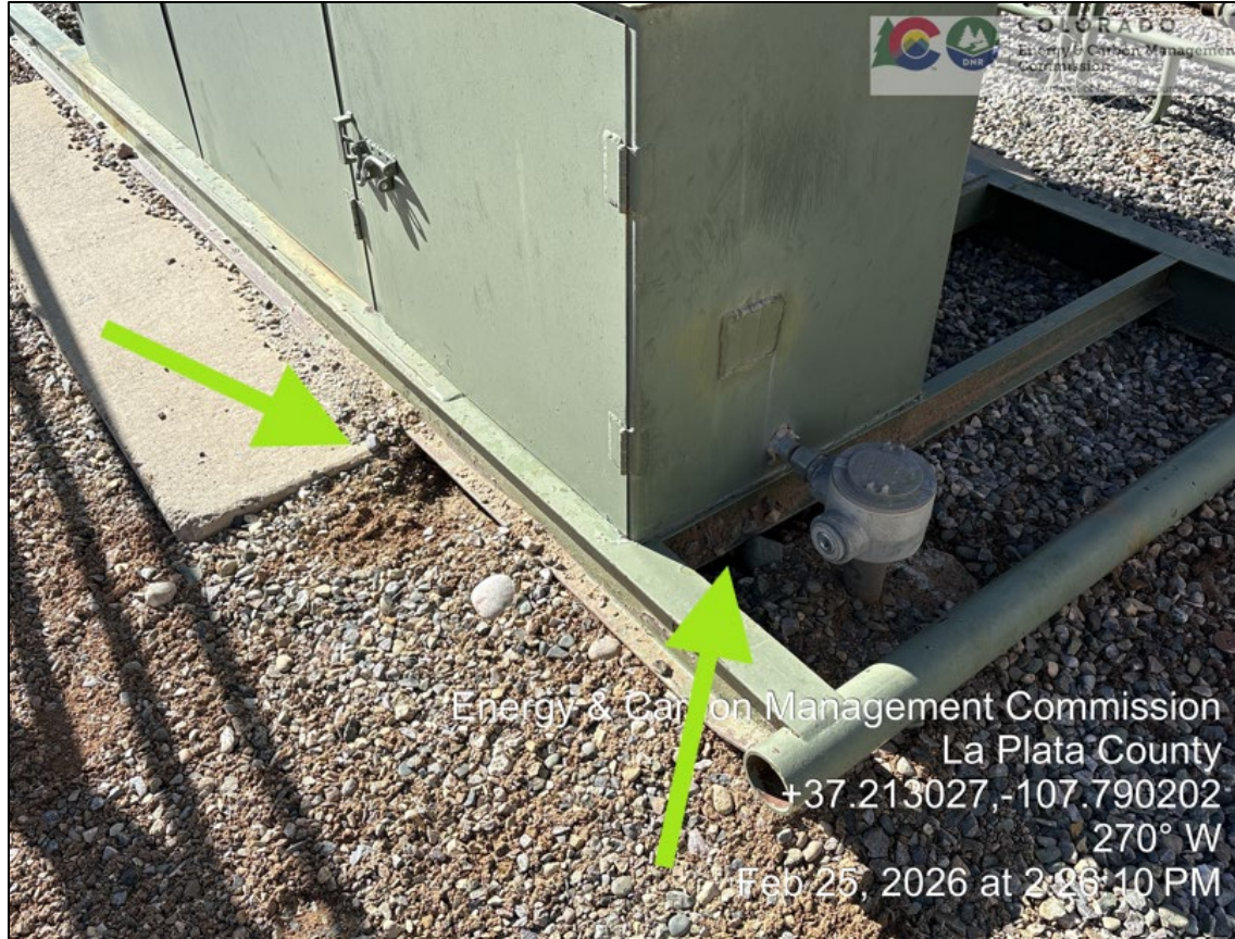
19. Wildlife burrows beneath Hester 2 horizontal heated separator structure.
