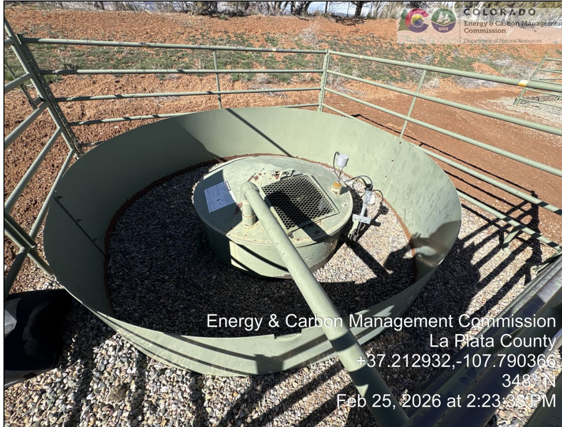
16. Hester 2 21 BBL produced water w. natural gas tank and secondary containment.
