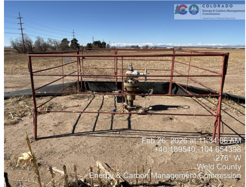
Photo 2 well head and equipment
