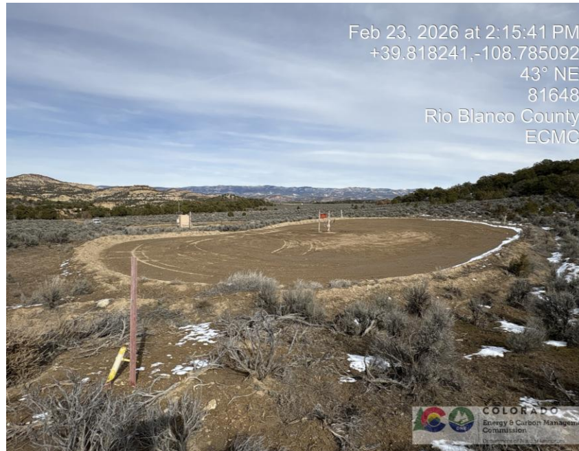
Photo # 2327 SW corner of location
