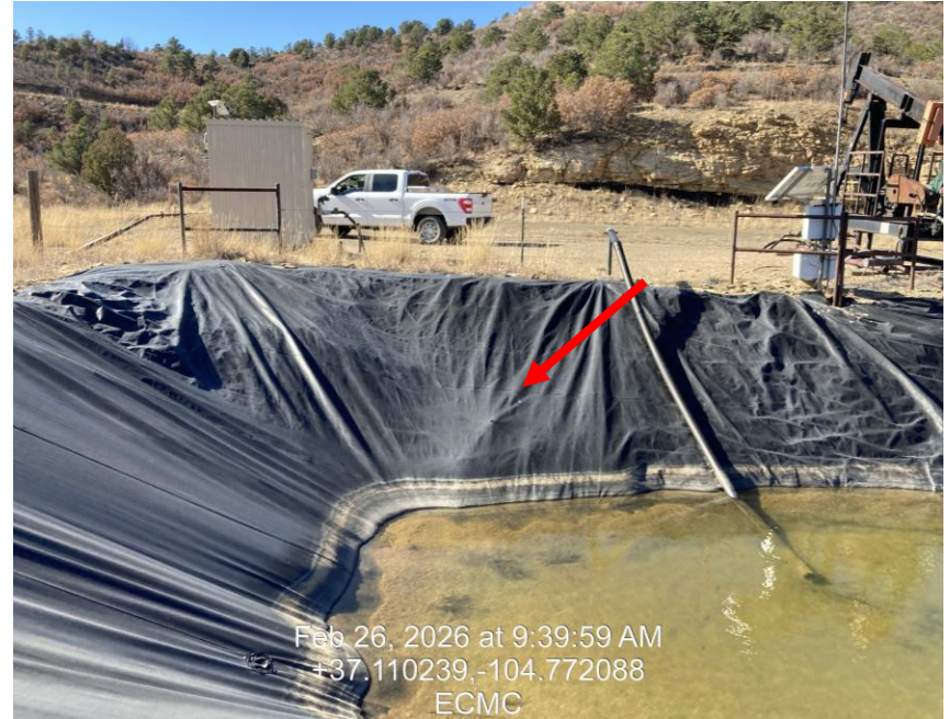
Photo 6: Hole in pit liner
