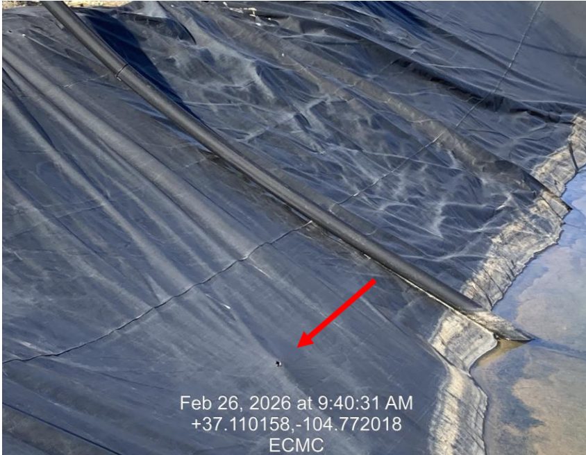
Photo 5: Hole in pit liner
