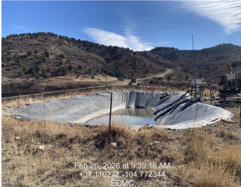
Photo 3: Pit Facility ID 261259
