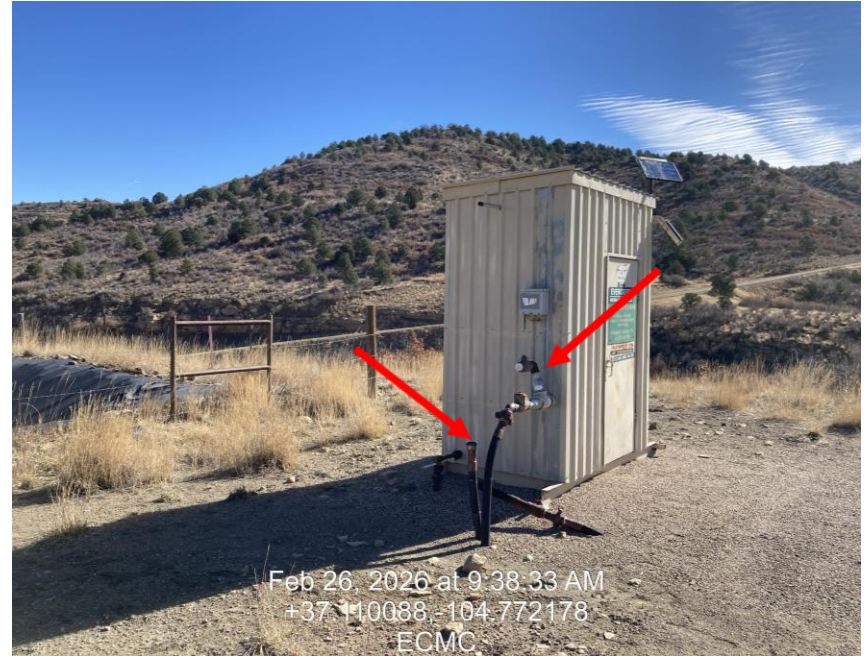
Photo 4: Meter house, disconnected flowlines
