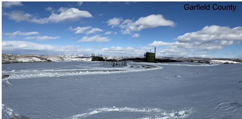
South West corner of location.
