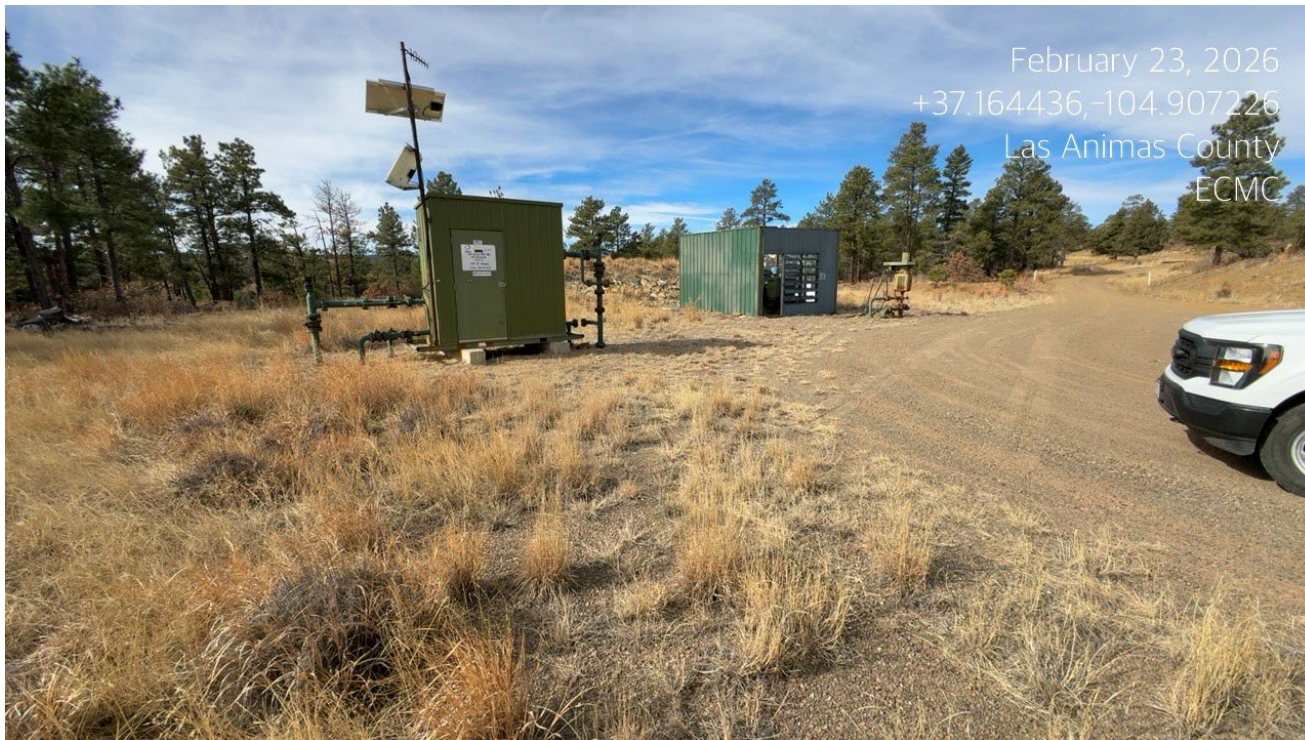
Photo 2. Well sign is posted at meter shed.
