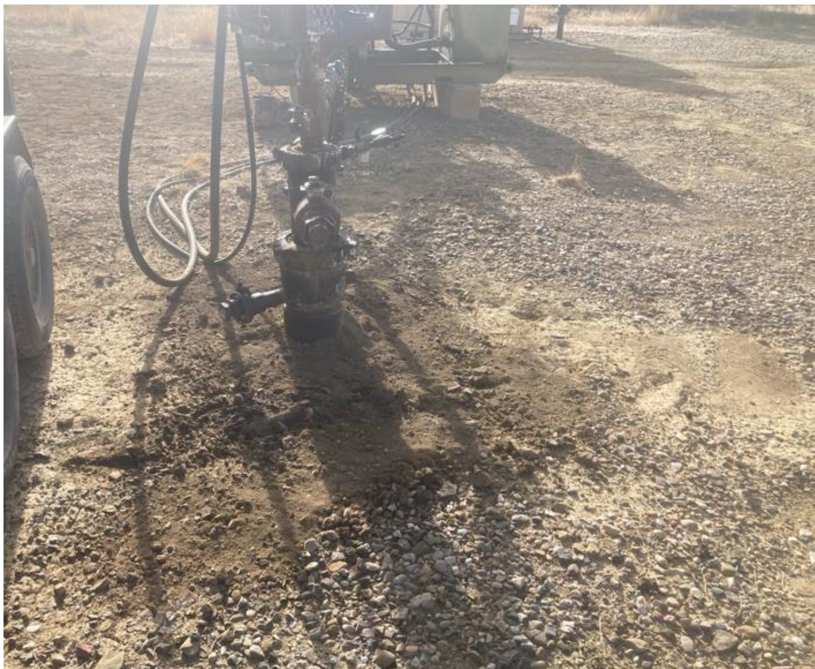
PHOTO 1: THE LEAK HAS BEEN STOPPED ON THE WELL HEAD AND PACKING HAS BEEN TIGHTENED. THE IMPACTED SOIL HAS BEEN REMOVED FROM LOCATION AND REPLACED WITH FRESH PAD MATERIAL.
