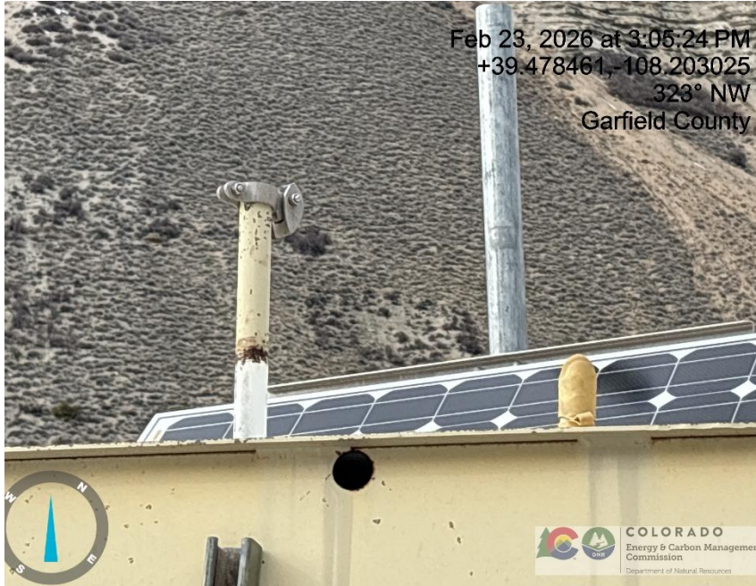
Photo # 2804 PRV vent line does not comply with CECMC pressure safety device rules
