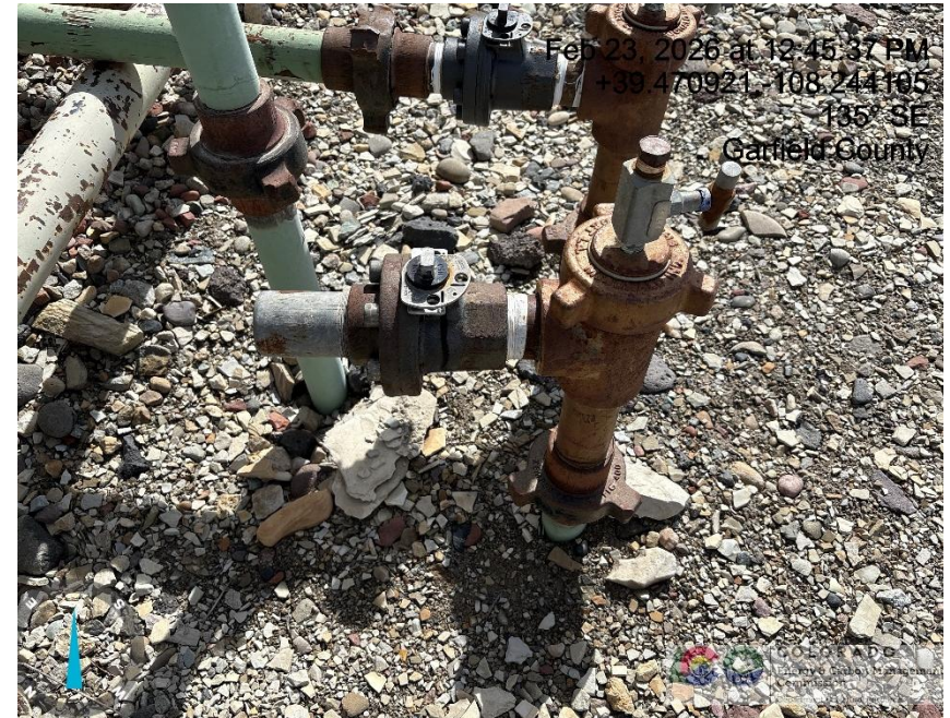
Photo # 2342 Unused flowline lacks lockout tagout (OOSLAT)
