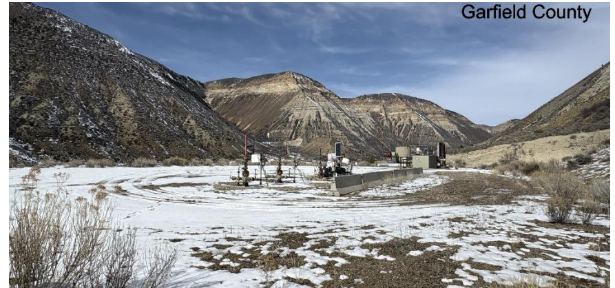
South East corner of location.
