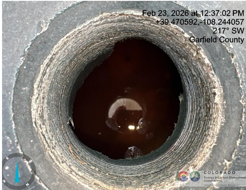
Photo # 2343 Failure to maintain chemical BMP – Chemical tank containment approximately 3/4 full of fluid/BMP not sufficient to contain possible spill
