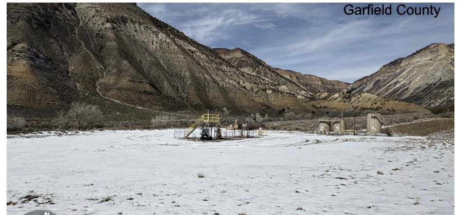
South East corner of location.
