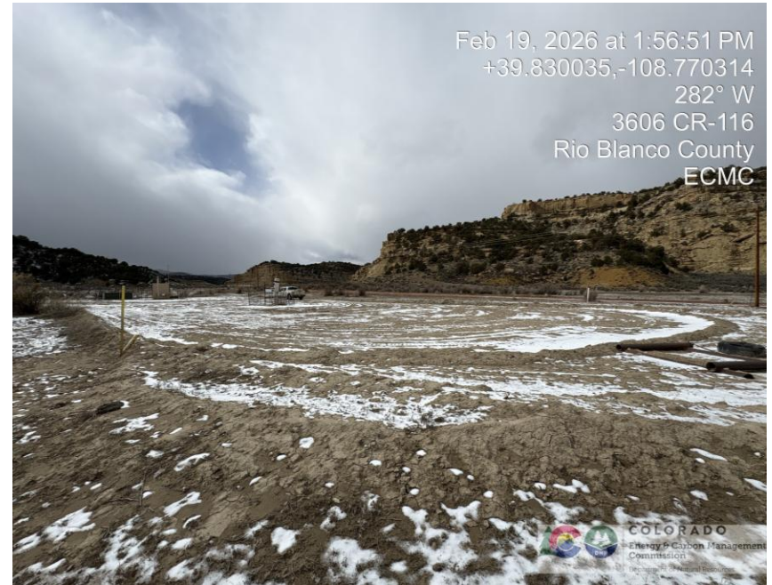
Photo # 2213 SE corner of location
