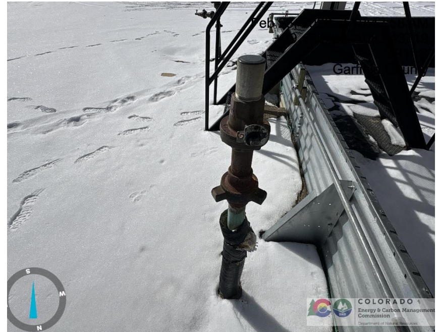
Photo # 1570 Unused flowline lacks lockout tagout (OOSLAT)
