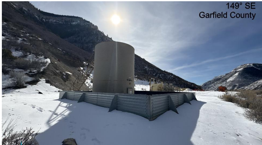
North West corner of location.
