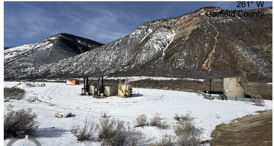
North East corner of location.
