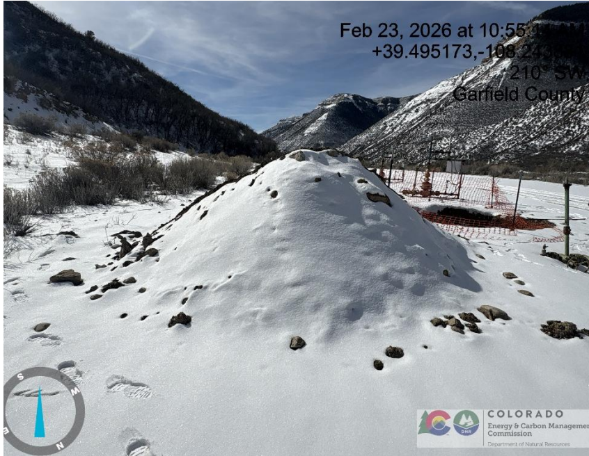
Photo # 1573 Soil stockpile lacks BMP's
