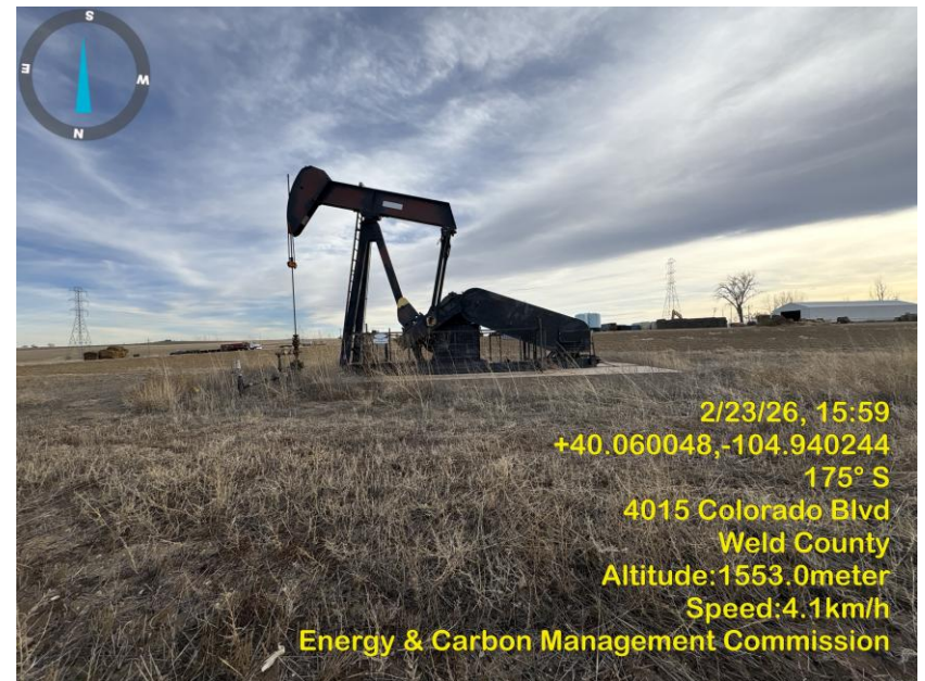
Photo 8 Tall dead vegetation around the wellsite.
