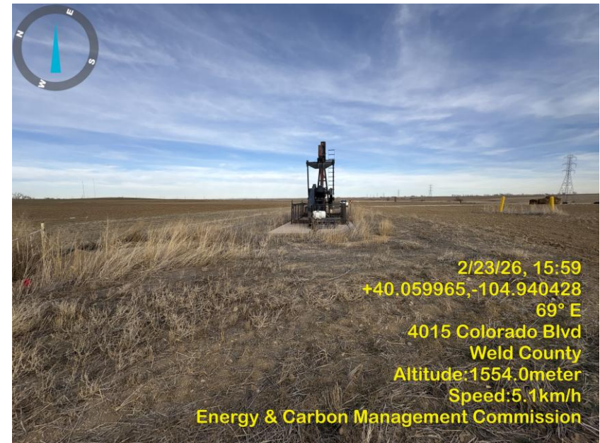
Photo 6 Tall dead vegetation around the wellsite.
