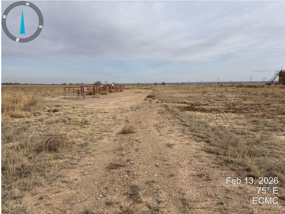
Photo 1. Looking east down the access road across the well area. Desirable perennial vegetation appears to be progressing in the interim area. Tumbleweed is present touching equipment.
