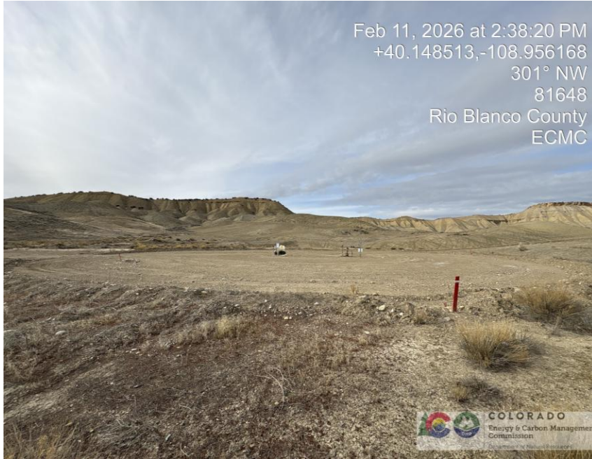
Photo # 2107 SE corner of location
