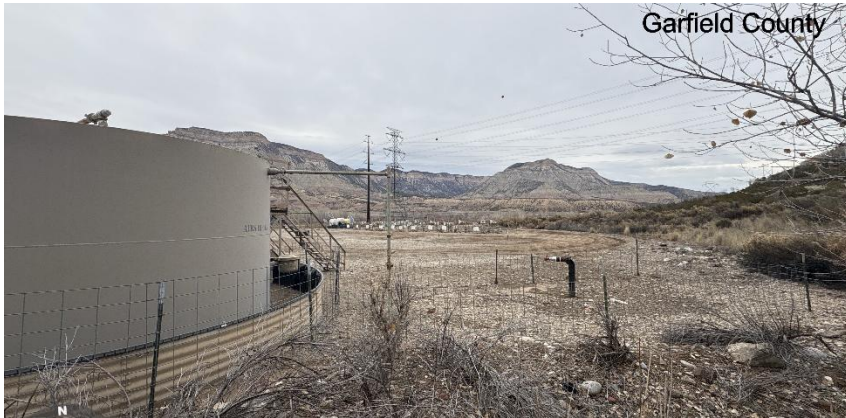
South West corner of location.
