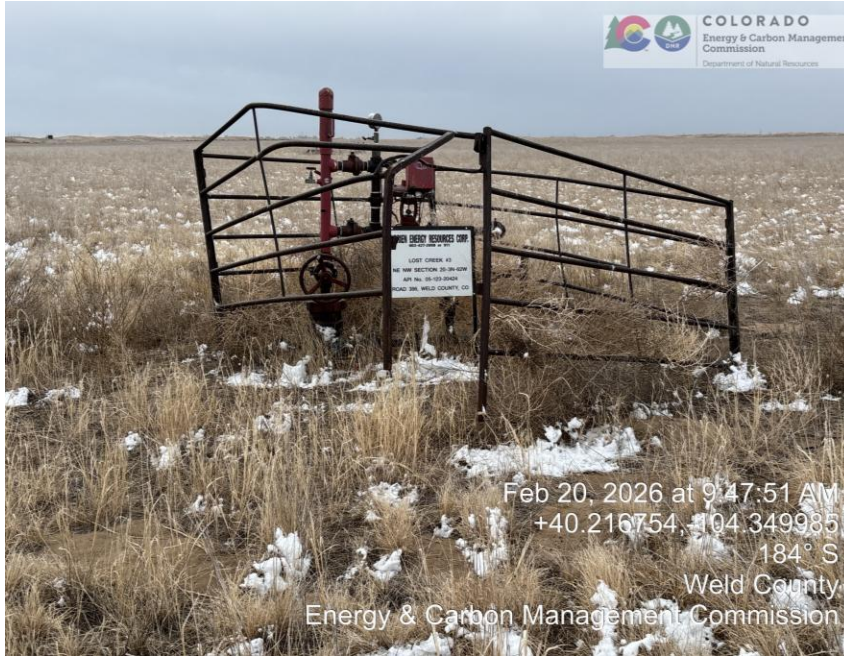
Photo 1 well head and equipment
