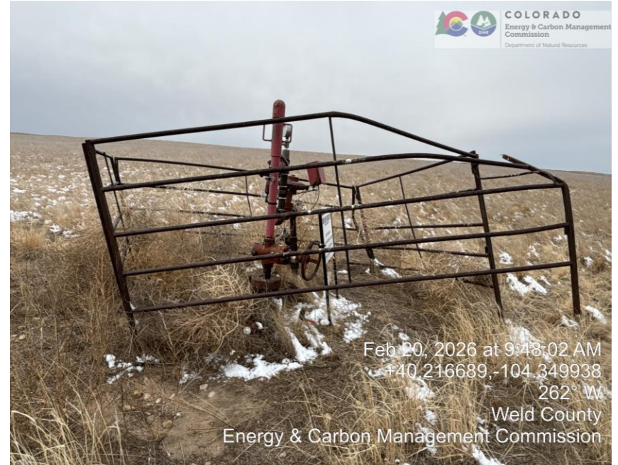
Photo 2 well head and equipment
