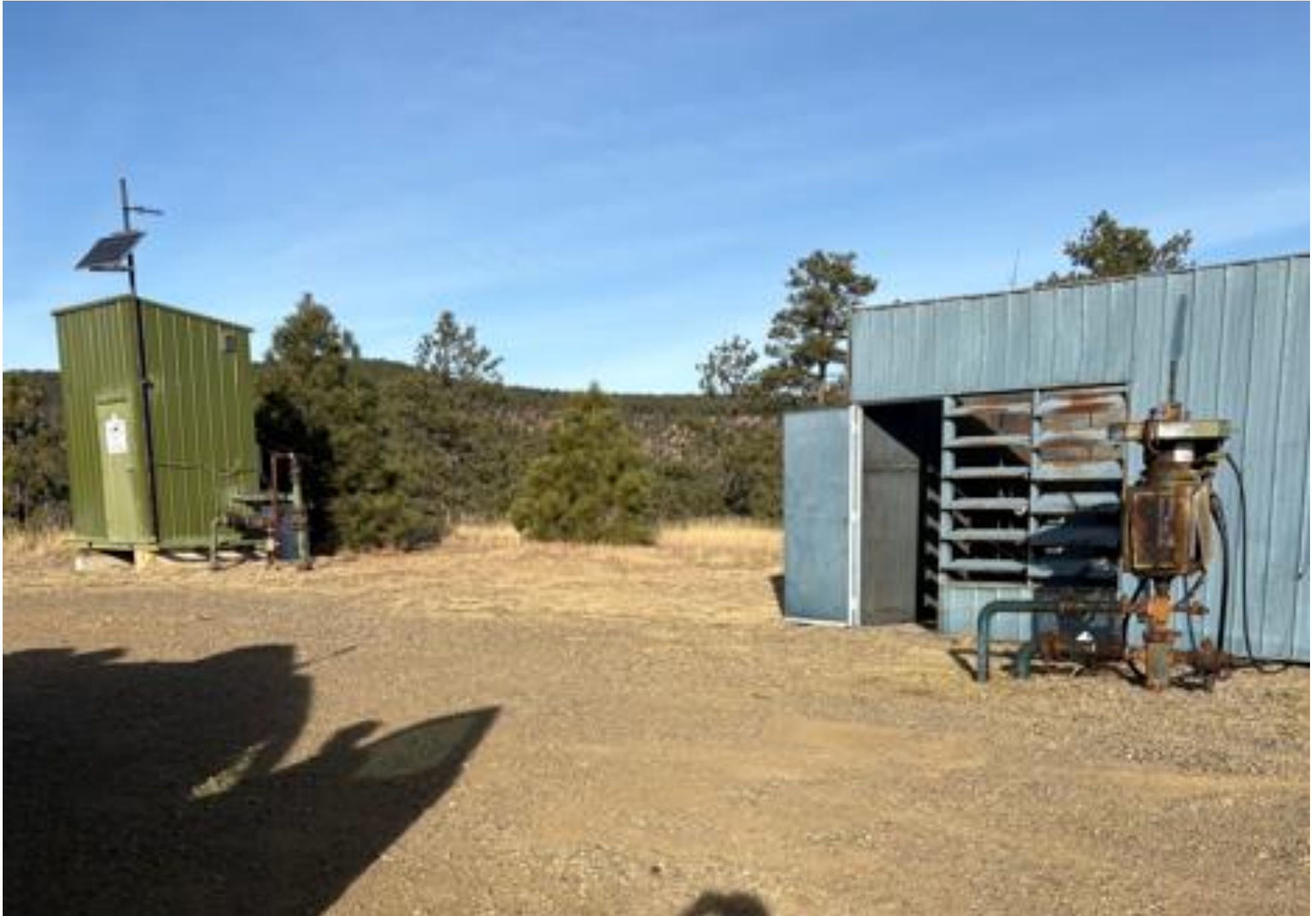
PHOTO 1: ALL VEGETATION HAS BEEN CUT AND REMOVED AROUND THE OPERATING EQUIPMENT.
