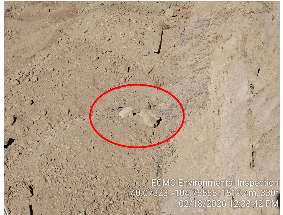
Photo 6 – Cement used in backfill in open excavation.
