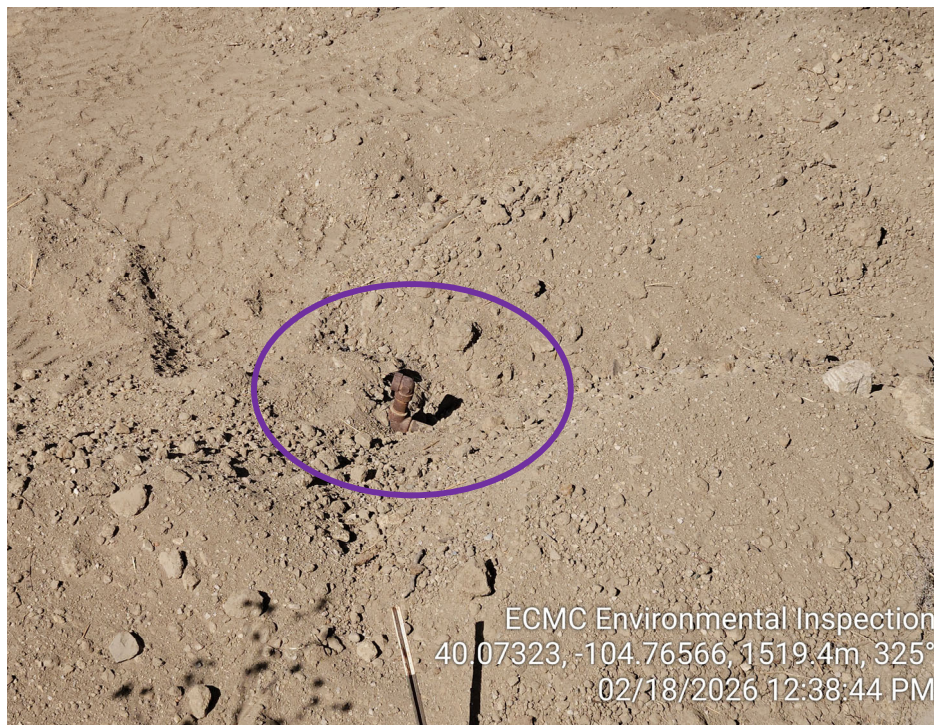
Photo 7 - Uncapped pipe in open excavation.
