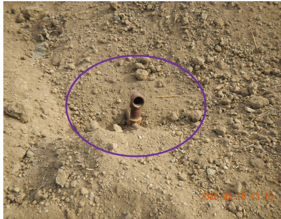
Photo 8 - Uncapped pipe in open excavation.
