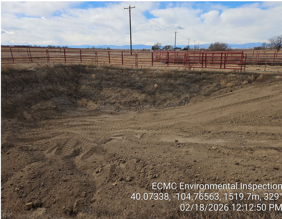
Photo 3 - Open excavation; excavation has been partially backfilled
