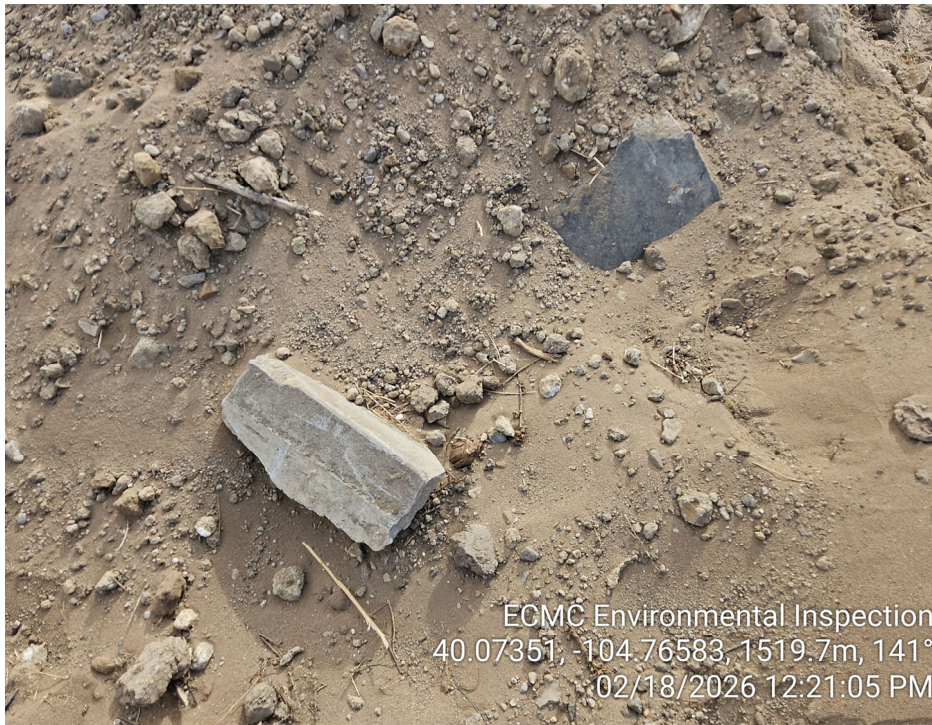
Photo 15 - Soil stockpiles on location for backfill; concrete present in backfill
