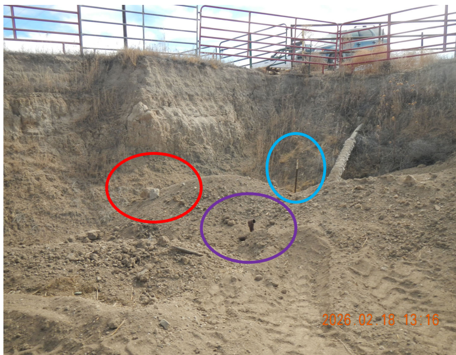
Photo 9 - Cement in backfill in open excavation (red). Uncapped pipe (purple) and t-post (blue) present in open excavation.
