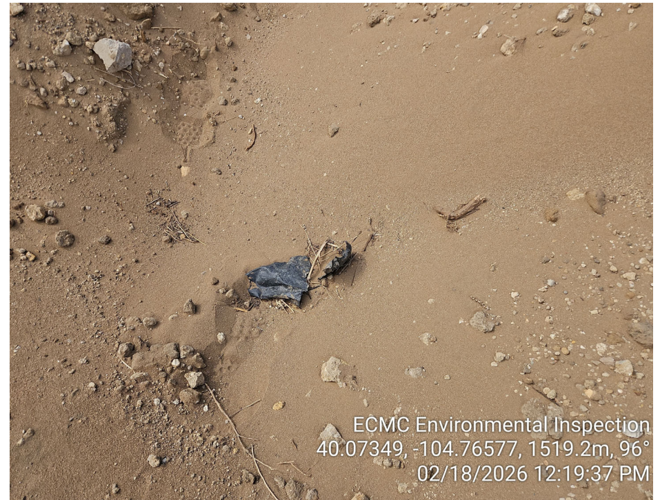
Photo 12 - Soil stockpiles on location for backfill; trash present in backfill
