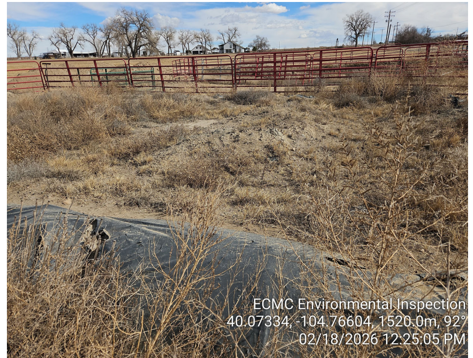
Photo 18 – Area of previously stockpiled contaminated soil; a small amount of soil remains within the stockpile. “Contaminated” marker and liner still present. Holes in liner visible. Weeds throughout.
