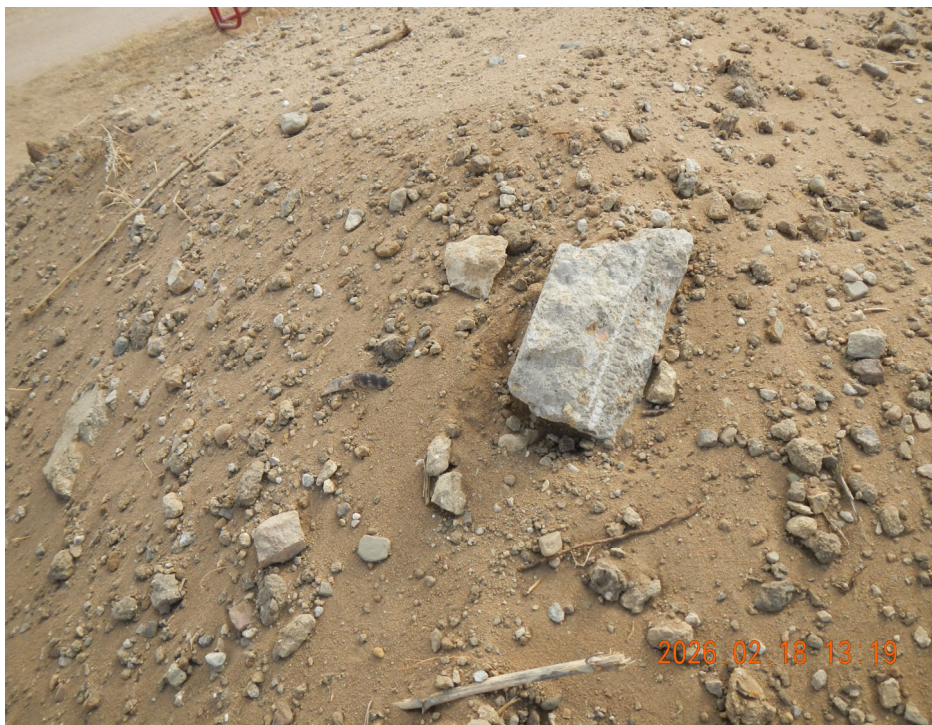
Photo 13 - Soil stockpiles on location for backfill; concrete present in backfill
