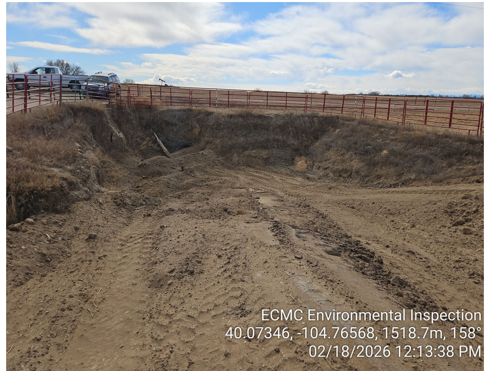
Photo 4 - Open excavation; excavation has been partially backfilled
