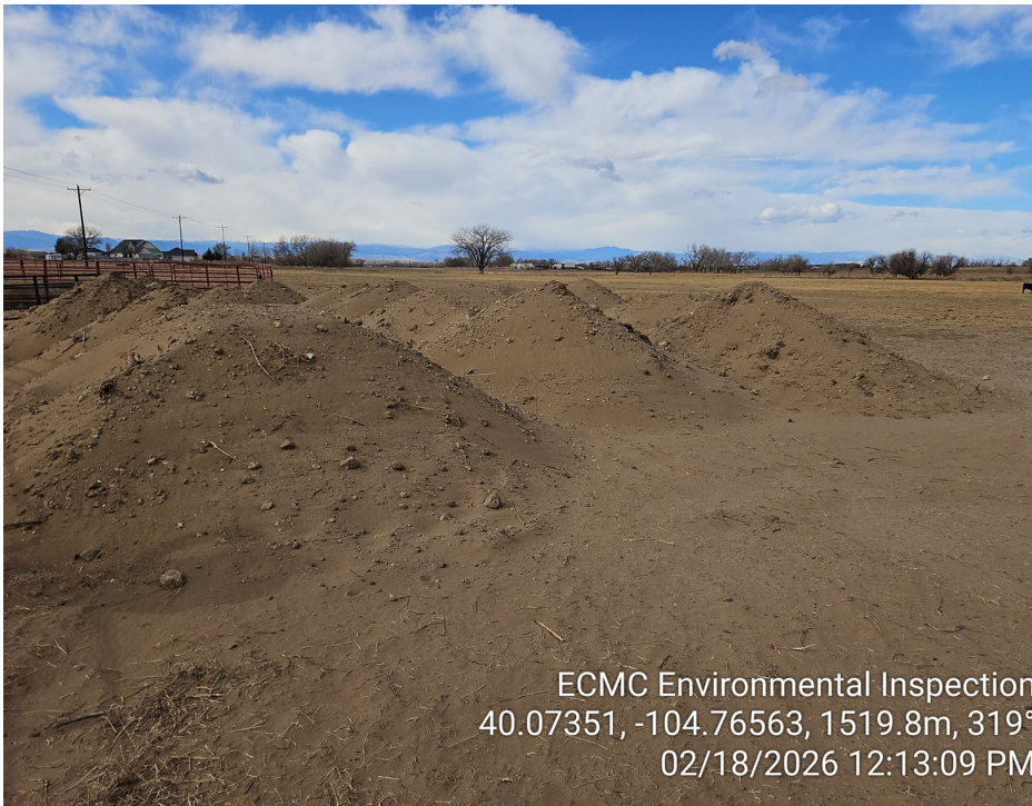
Photo 11 - Soil stockpiles on location for backfill
