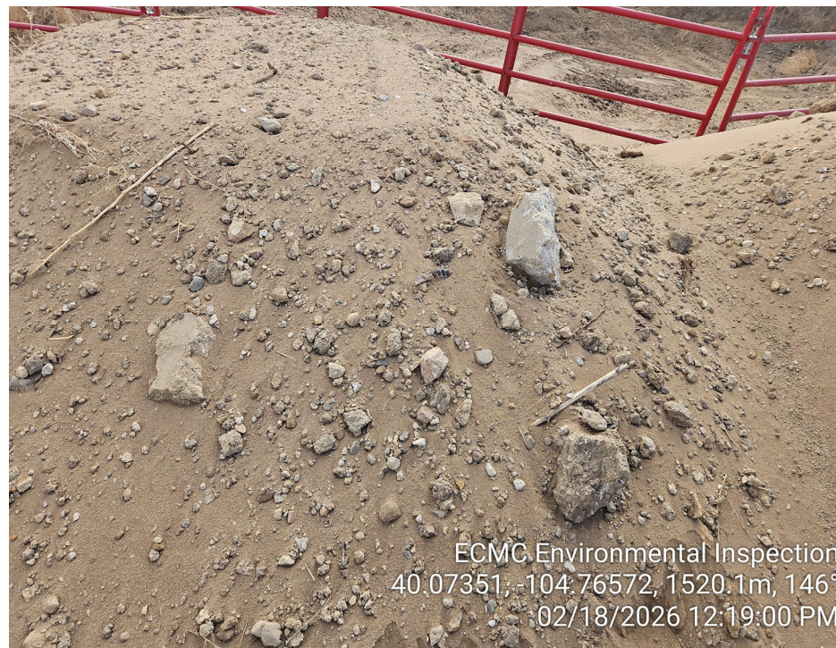
Photo 14 - Soil stockpiles on location for backfill; concrete present in backfill
