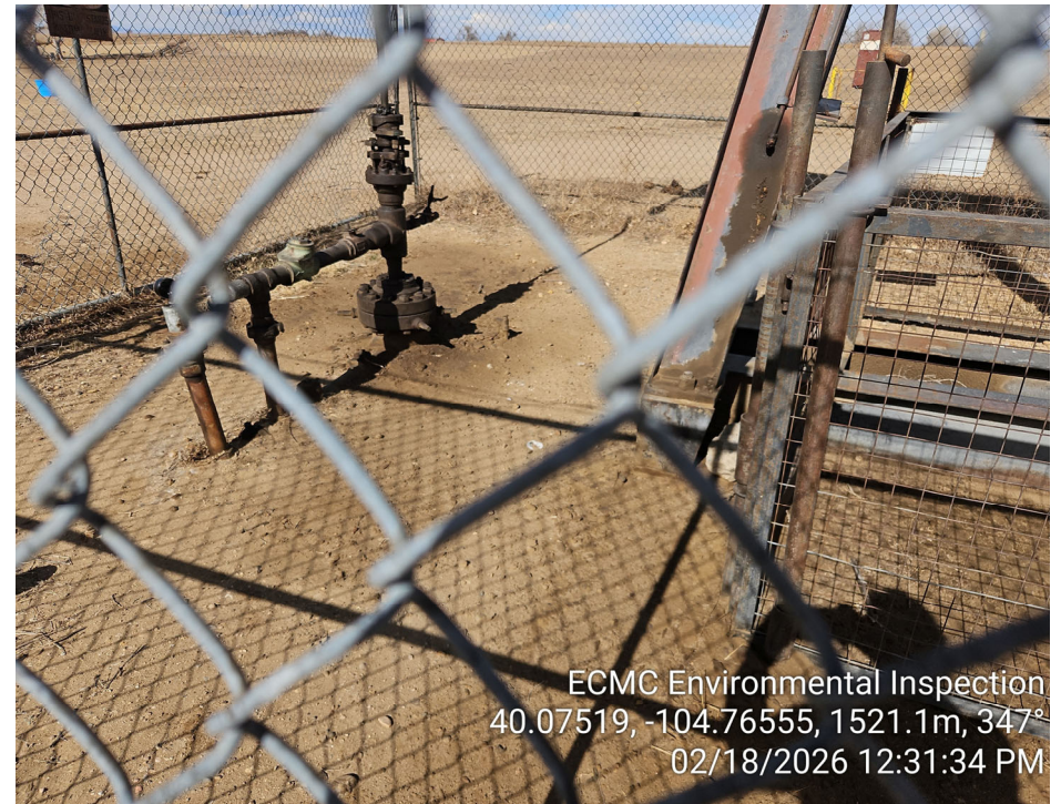
Photo 22 - UPRR 50 Pan Pam D#1 wellhead. Stained soil at wellhead and surrounding area.
