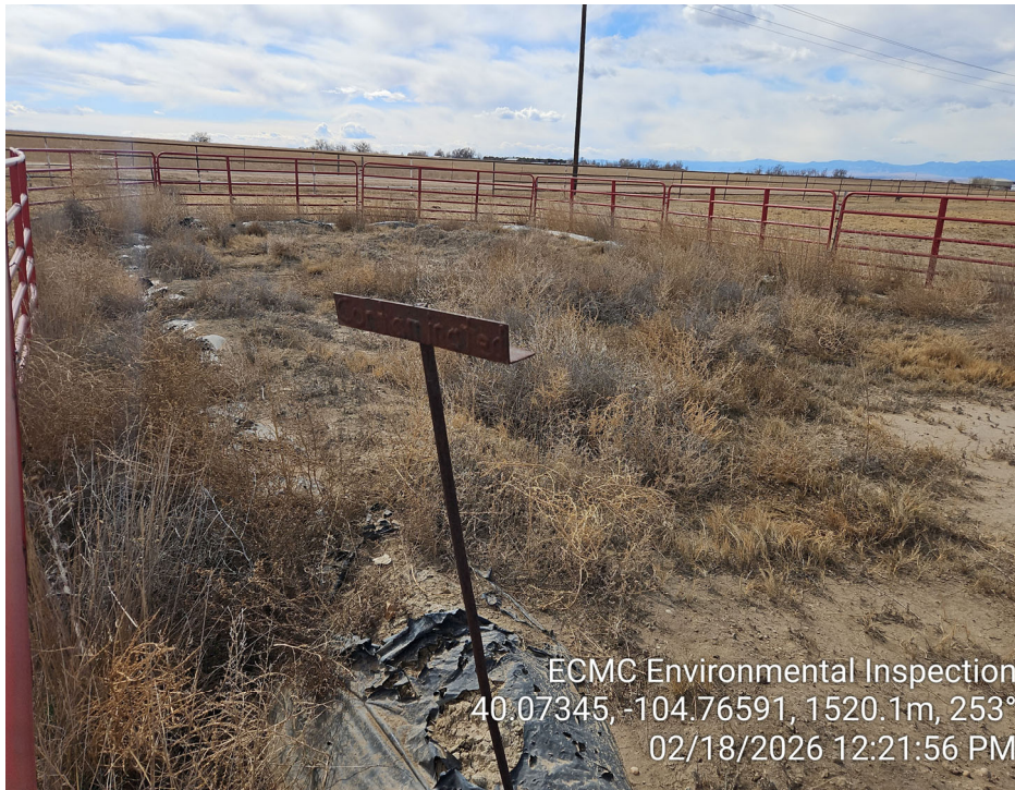
Photo 17 – Area of previously stockpiled contaminated soil; a small amount of soil remains within the stockpile. “Contaminated” marker and liner still present. Holes in liner visible. Weeds throughout.
