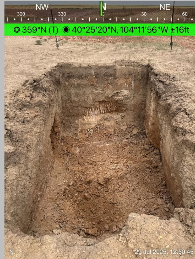
Excavation Looking North
