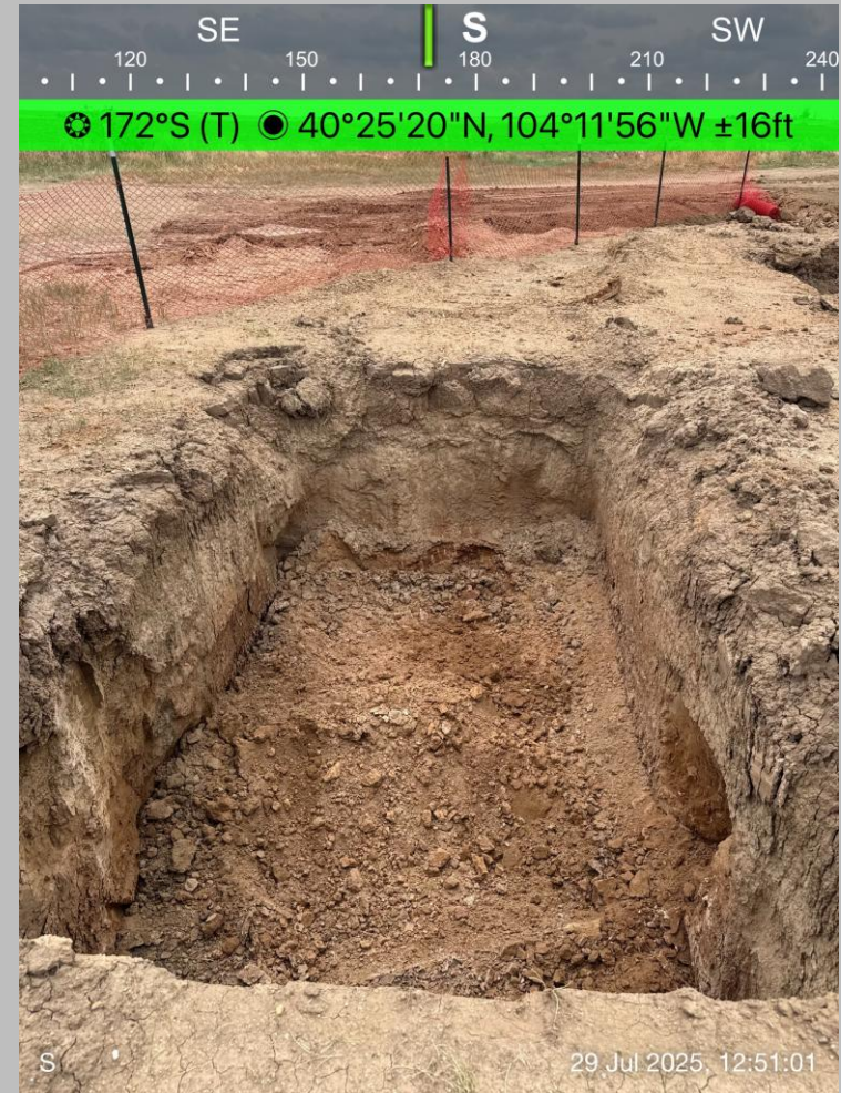
Excavation Looking South
