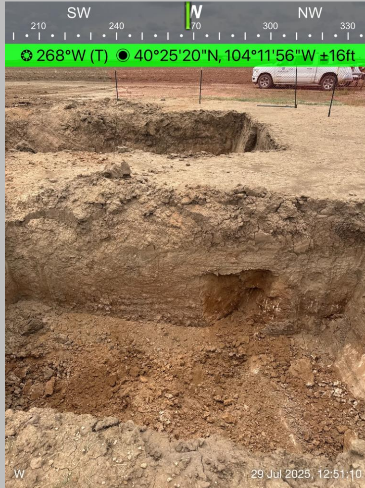
Excavation Looking West
