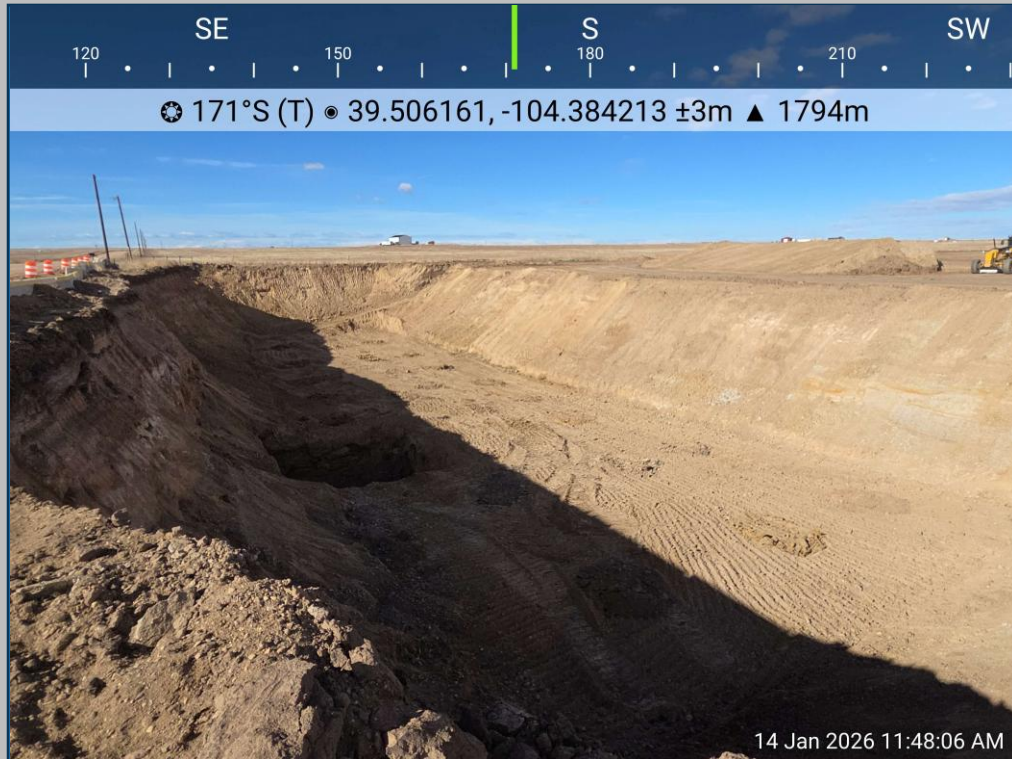
Excavation facing Northwest
