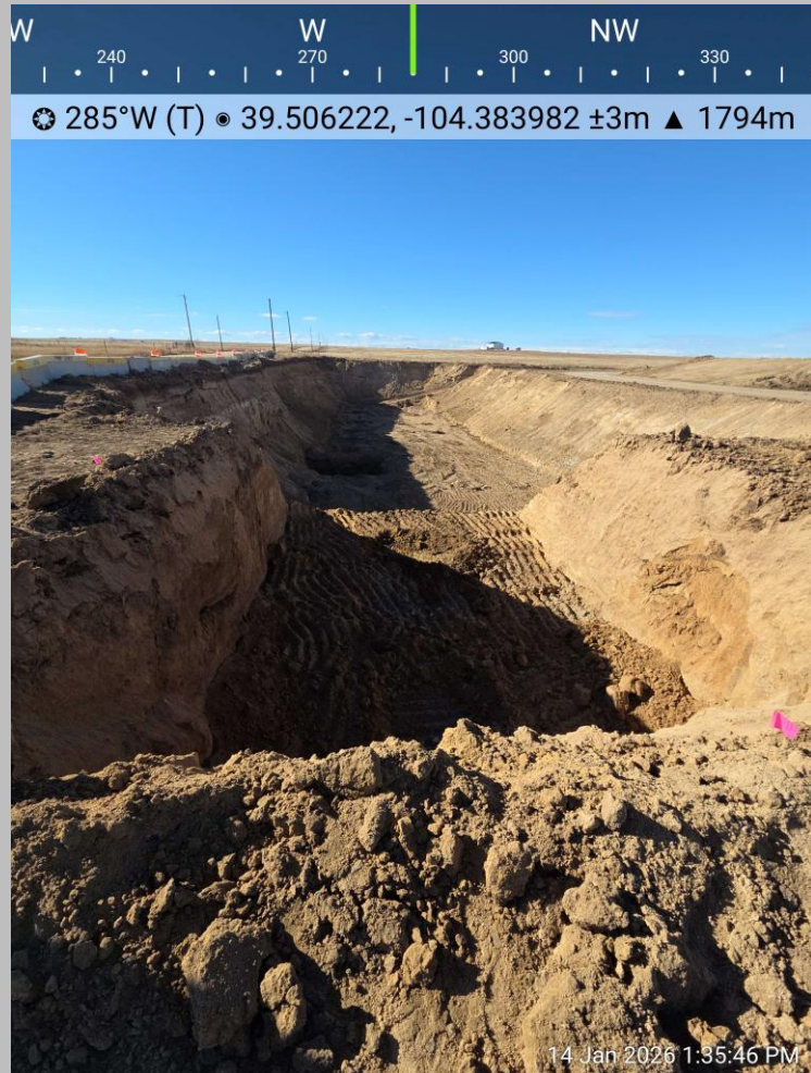
Excavation Facing West
