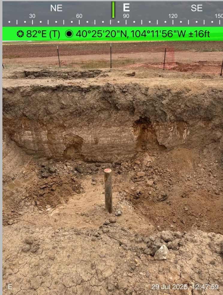
Excavation Looking East
