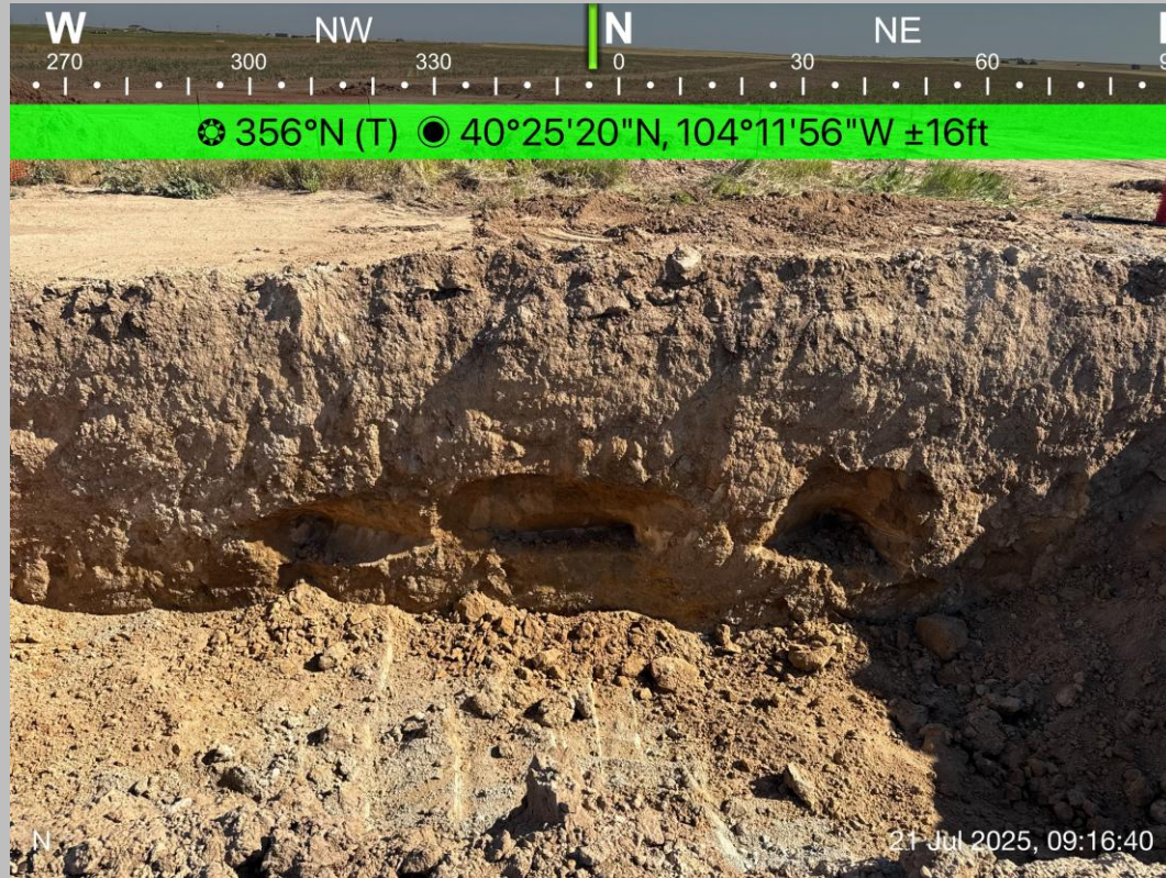
Excavation Overview Facing North
