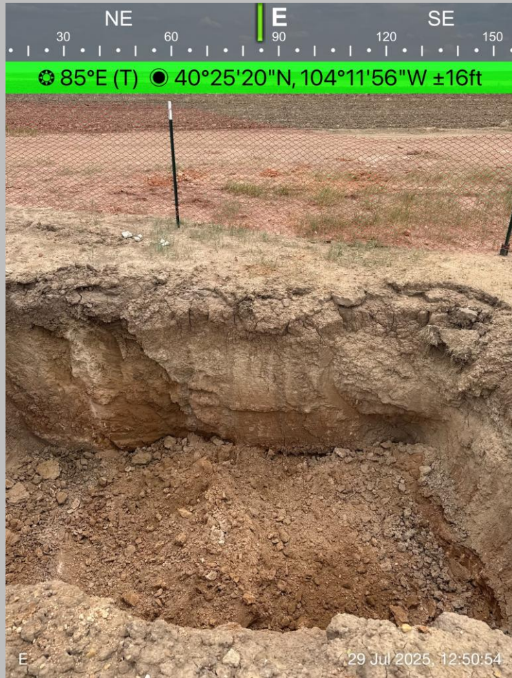
Excavation Looking East
