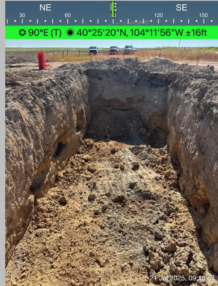
Excavation Overview Facing East
