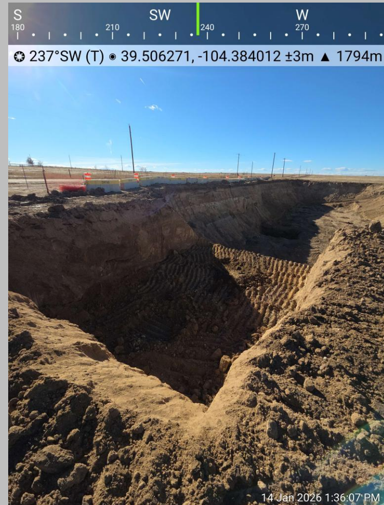
Excavation Facing Southwest
