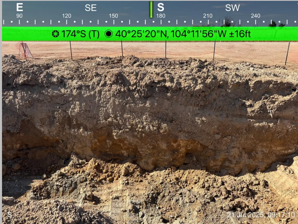
Excavation Overview Facing South
