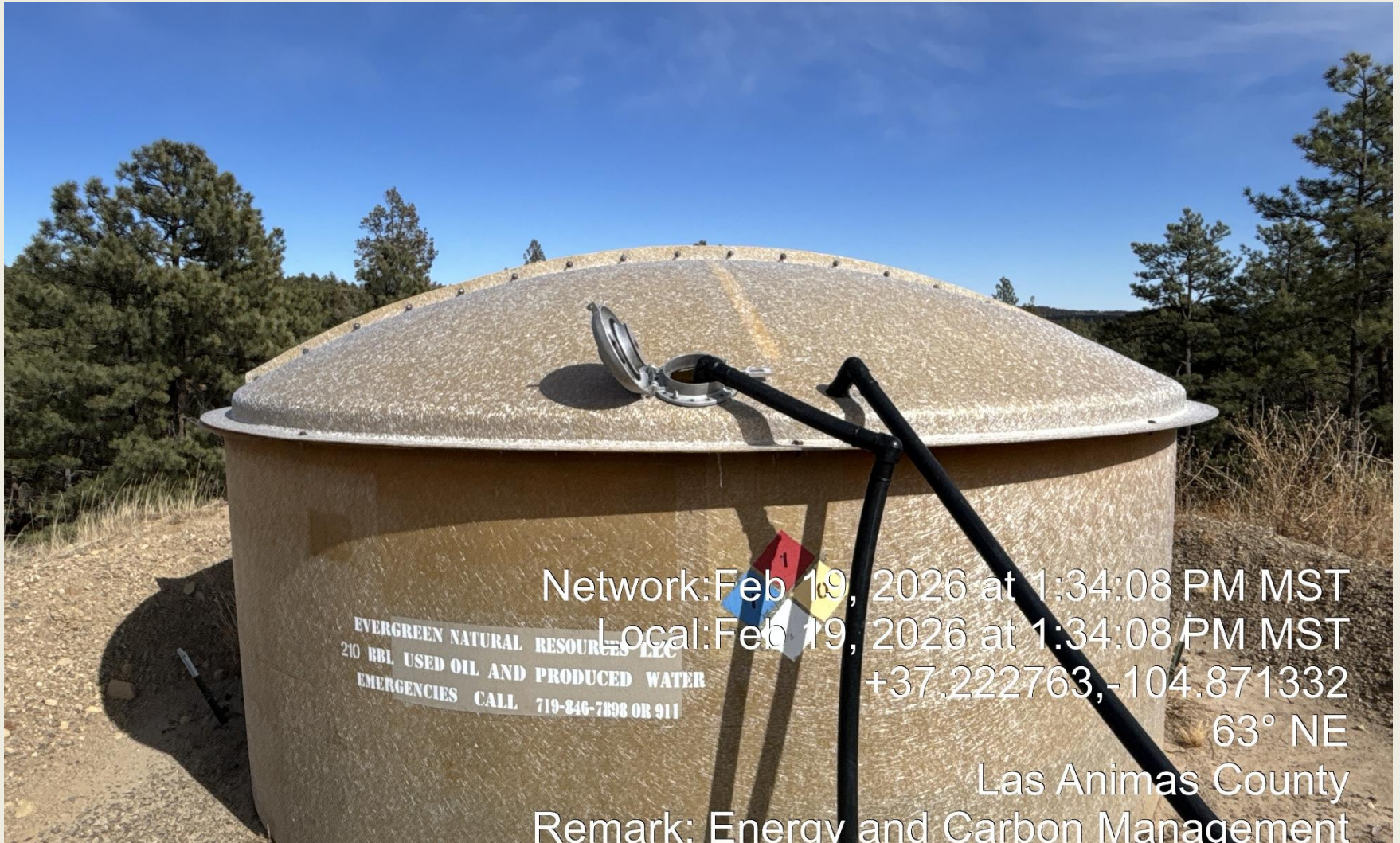
PHOTO 8: HATCH ON TANK IS OPEN WITH NO BIRD PROTECTION. PLUMB 2" PIPE SO HATCH CAN BE CLOSED OR INSTALL BIRD PROTECTORS PER RULE 608. CA DATE 3/3/2026.
