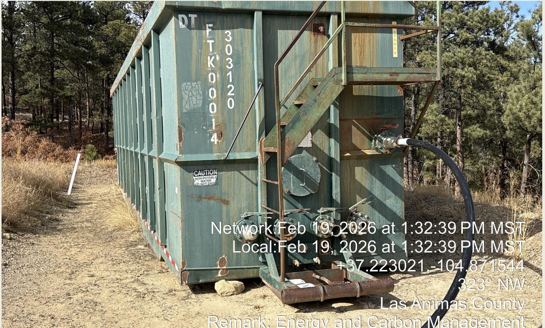
PHOTO 7: NO NFPA STICKER POSTED, NO CAPACITY POSTED AND CONTENTS IS PRODUCED WATER NOT NONE POTABLE WATER. REMOVE OR COVER NONE POTABLE WATER STICKER AND POST TANK BATTERY SIGHS PER RULE 605. CA DATE 3/3/2026.
