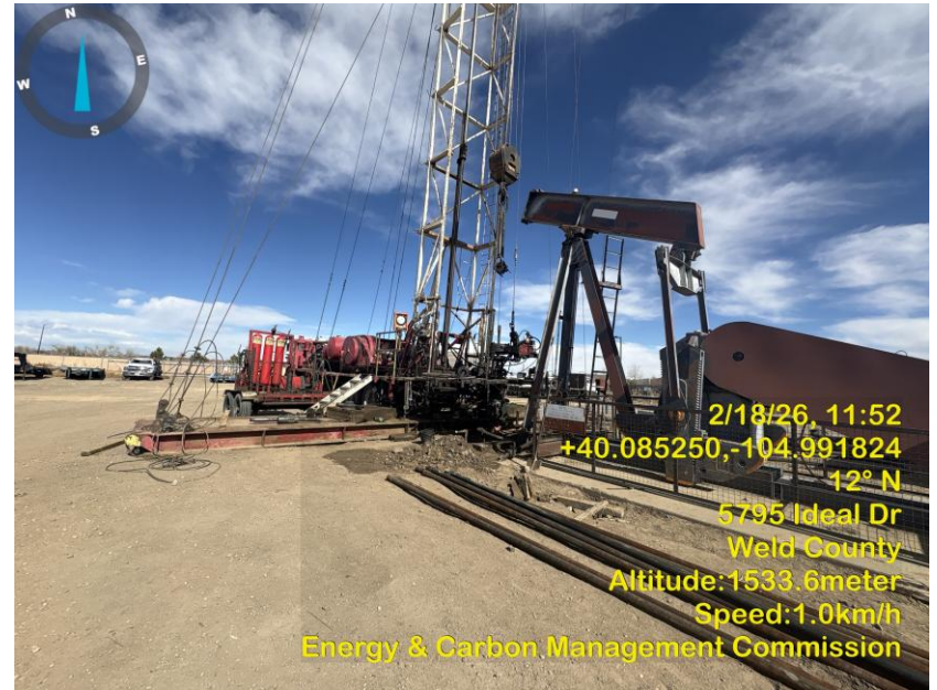
Photo 8 Rig floor, Pump jack.
