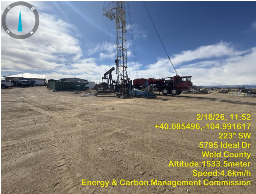
Photo 5 Rig pump, Rig.
