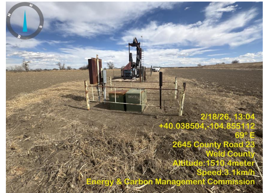
Photo 6 Unused Electric panel, meter box & transformers.
