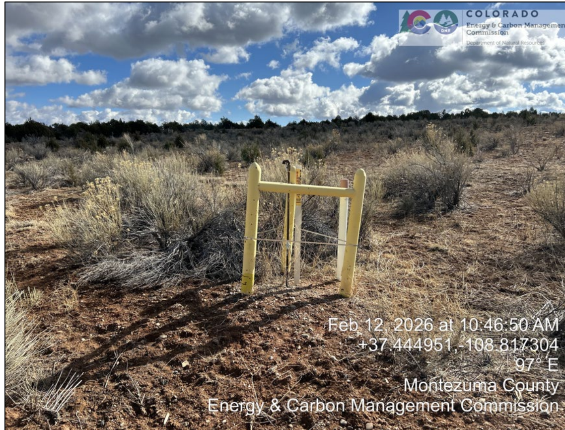
8. Annular vent behind pipe barricade.
