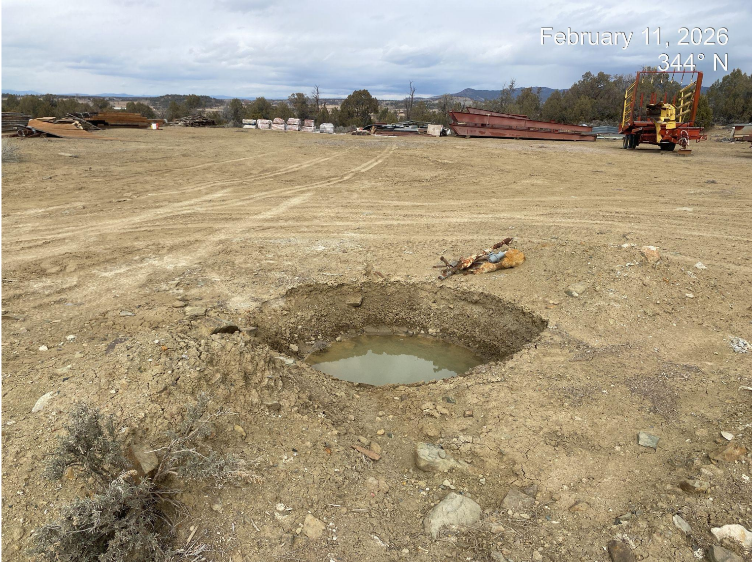
Photo 3. View of plugged well location. Pit remains with water and old piping reuipment.
