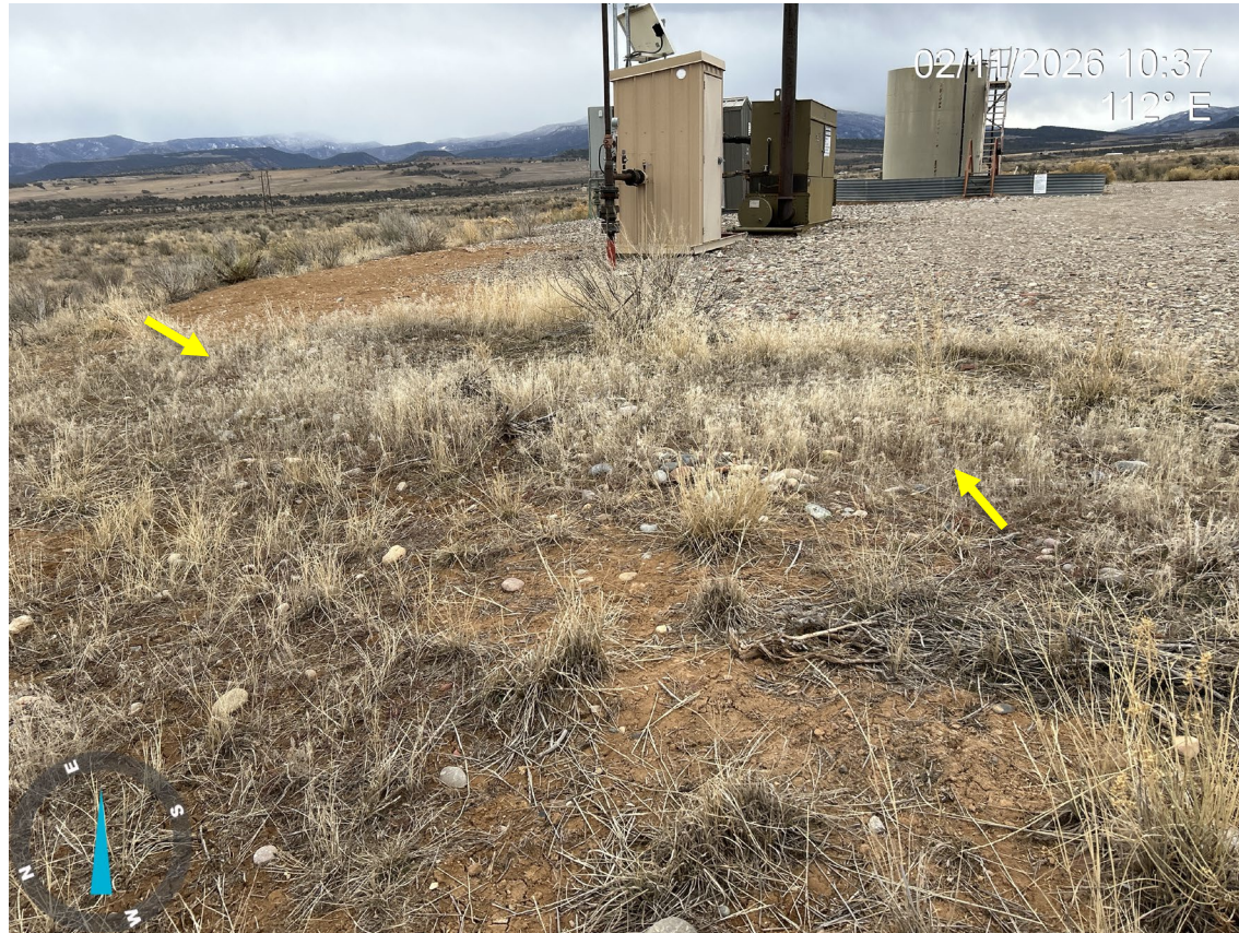
Photo 4: Photos showing cheatgrass (yellow arrow) is present around the margins of the working pad surface.
