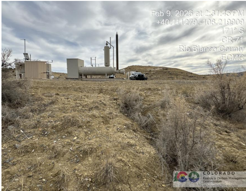
Photo # 1979 Failure to minimize erosion & transport of sediment off location/insufficient BMP's
