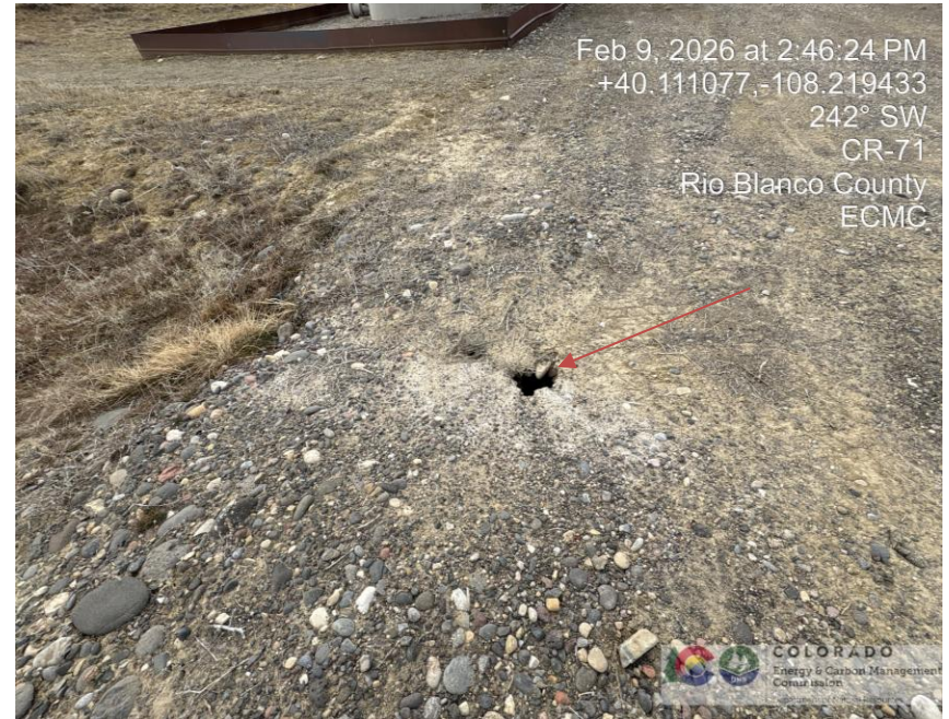
Photo # 1994 Tunnel erosion near entrance to location
