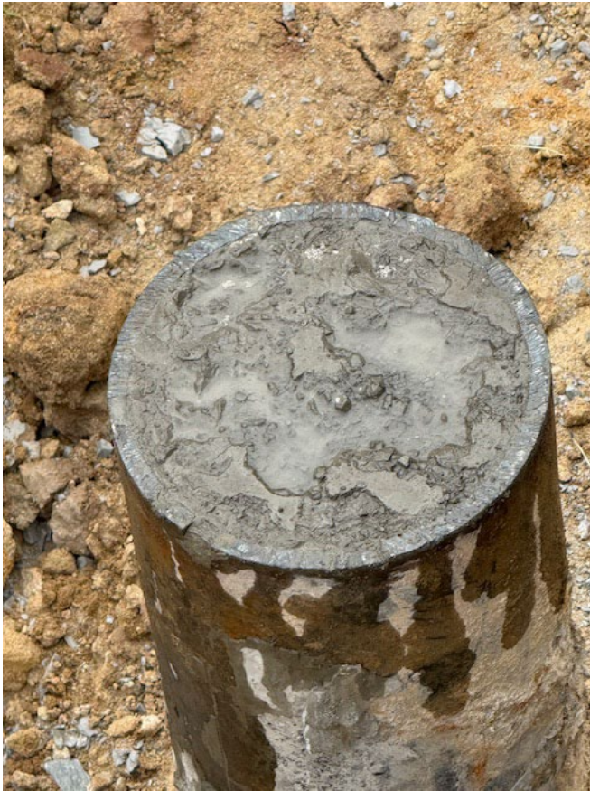
Casing Cut and Cement to surface
