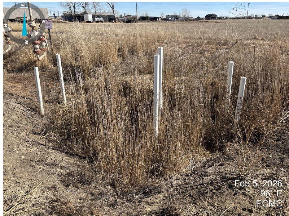
Photo 4. Looking east across the tank/ flowline reiser area. PVC pipes are present. A depression is present in the tank area.
