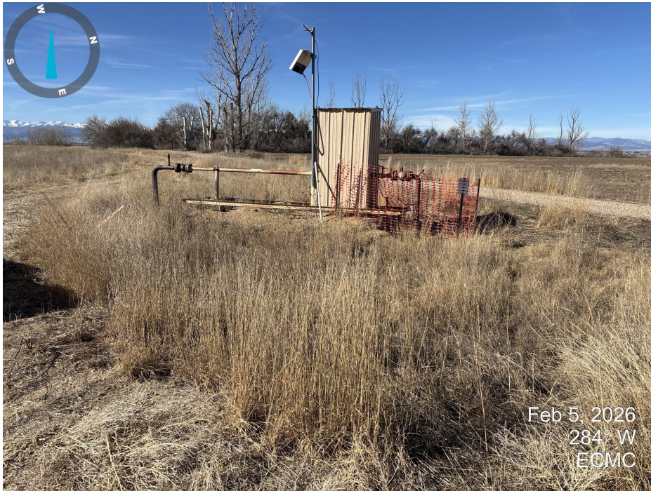
Photo 1. Looking west across the north part of the tank battery location. Meter shed and riser remains. Desirable perennial vegetation is present on the location. Undesirable weeds such as kochia are also present on the location.
