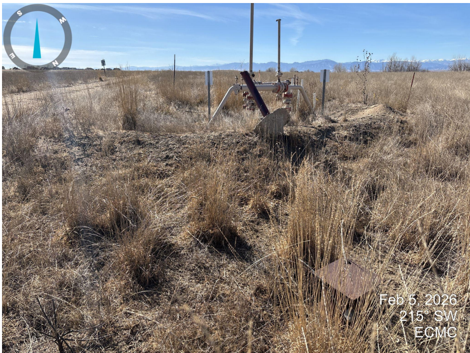
Photo 3. Looking south across the southern storage tank area. The large storage tank has been removed from the location. Pipe risers, pvc, and metal pipe remain on location.
