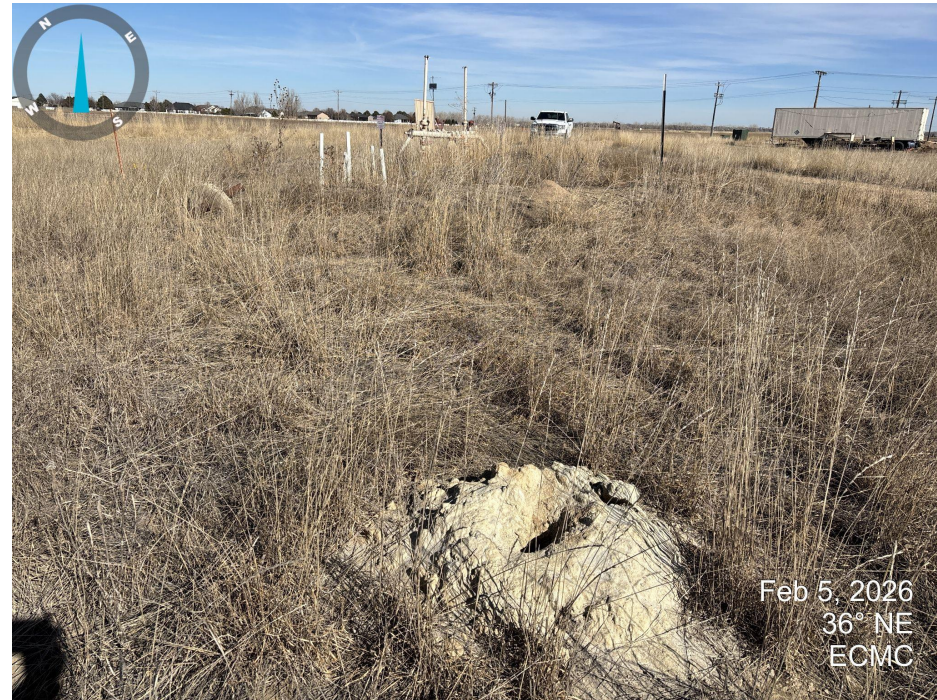
Photo 6. It appears that boreholes are present and open south of the tank battery location.
