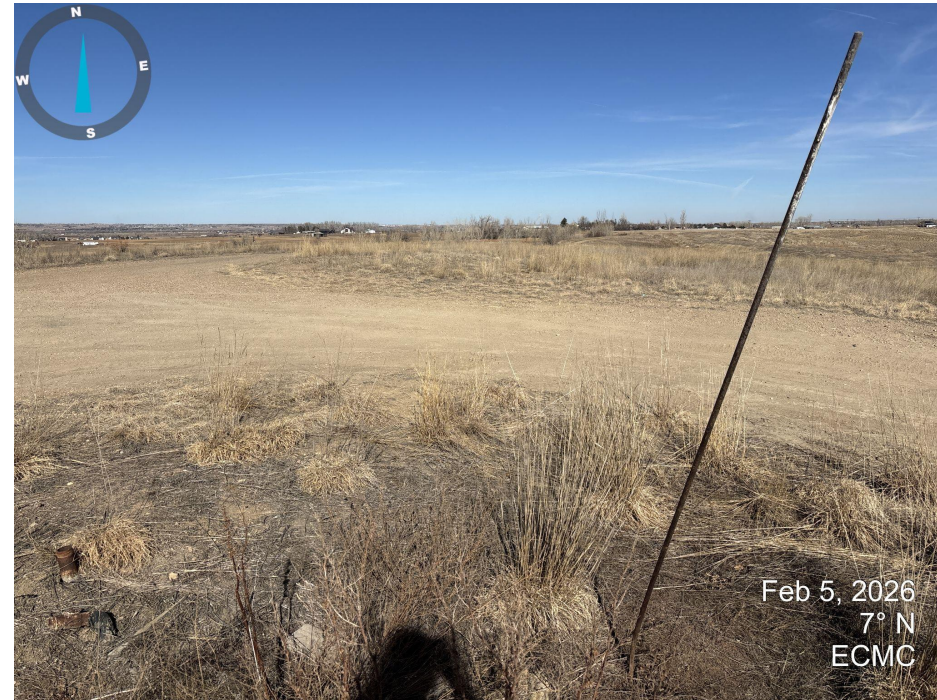
Photo 4. Looking north from the wellbore. Gravel remains on the location and the location size has not been reduced. It does not appear that reclamation was conducted on location.
