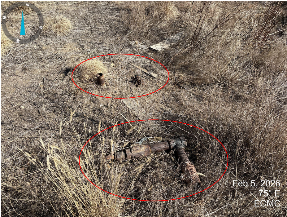
Photo 3. Oil and gas equipment and open pipe (red circle) remains on location.
