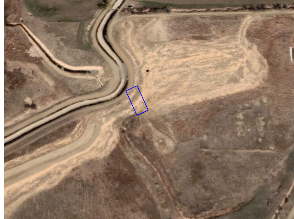
Photo 14. Google earth aerial imagery taken 04/2022. A stormwater ditch and basin unrelated to oil and gas was installed near the location. A 130' portion of the former access road (blue box) has been disturbed by non oil and gas activities.
