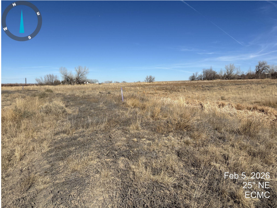
Photo 3. Ditch and detention pond.
