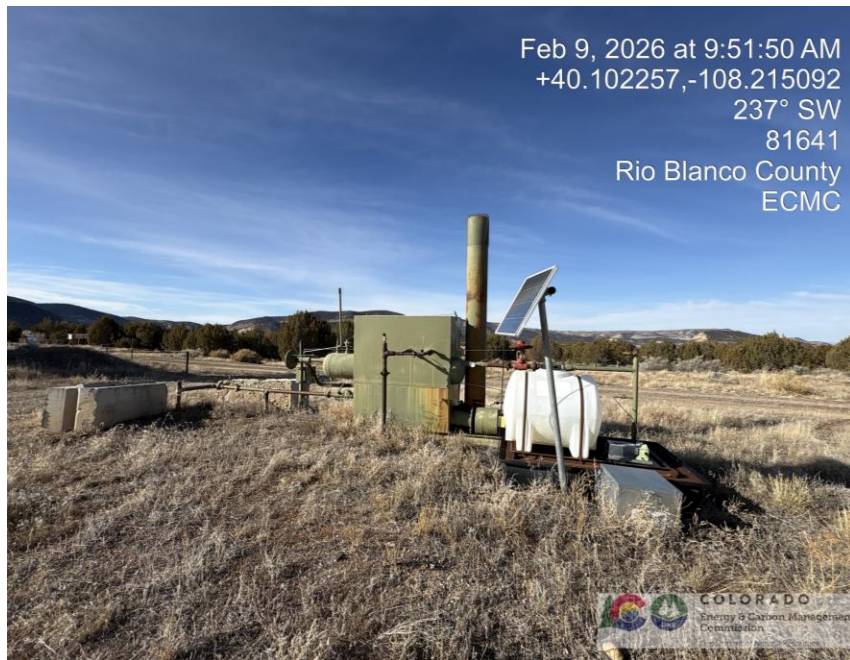
Photo # 1855 Weeds/undesirable plant species on location surrounding production equipment presents a potential fire hazard
