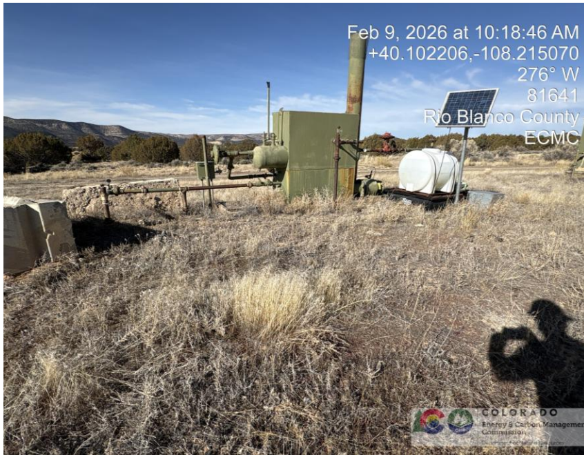
Photo # 1884 Weeds/undesirable plant species on location surrounding production equipment presents a potential fire hazard
