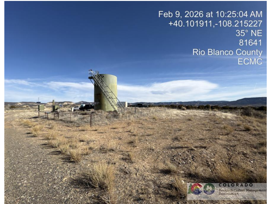
Photo # 1900 SW corner of location
