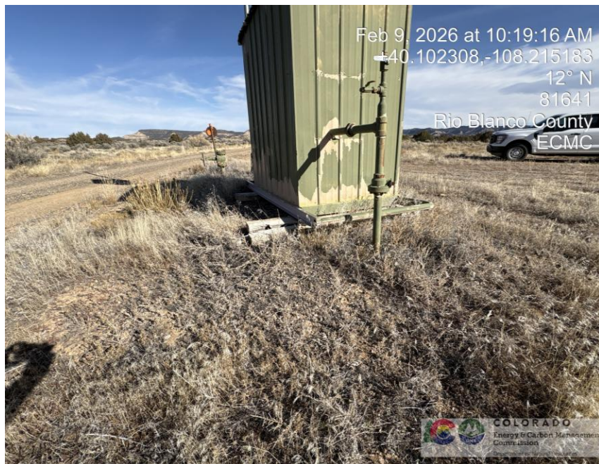
Photo # 1887 Weeds/undesirable plant species on location surrounding production equipment presents a potential fire hazard
