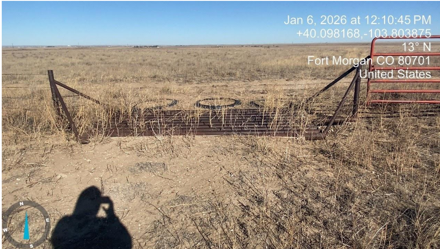
Photo 11. Photo shows cattle guard for access road has not been removed and large bare area present on access.
