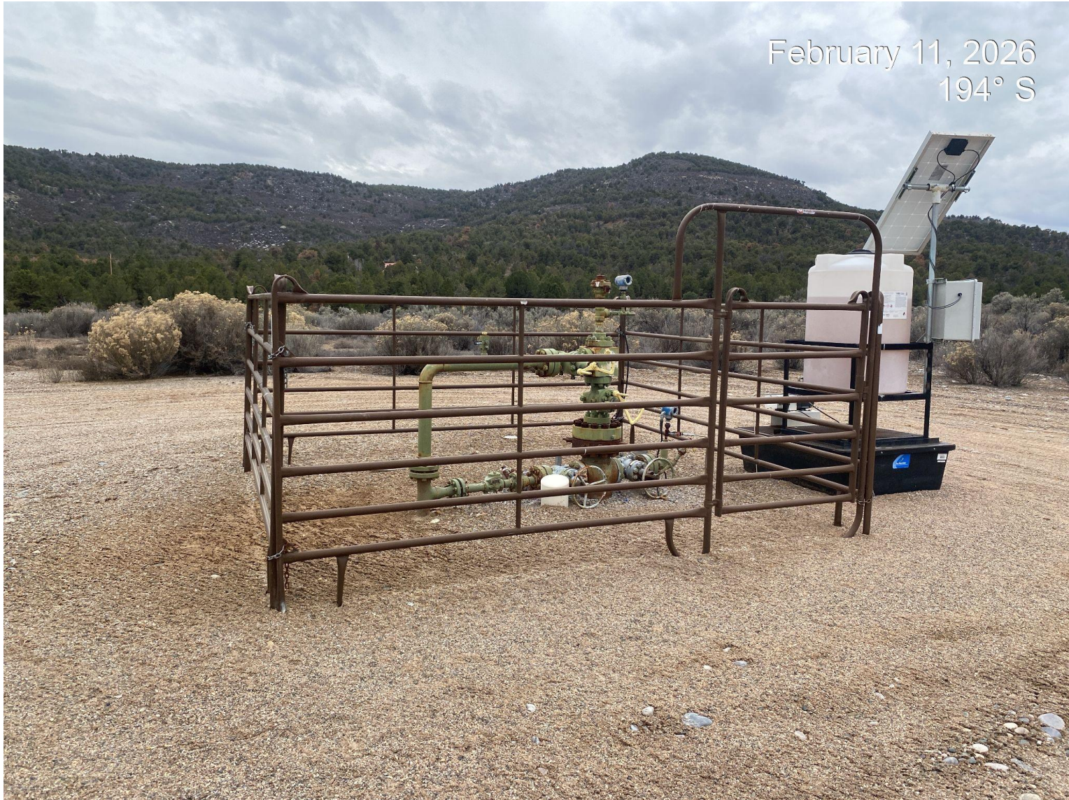
Photo 4. Wellhead assembly.
