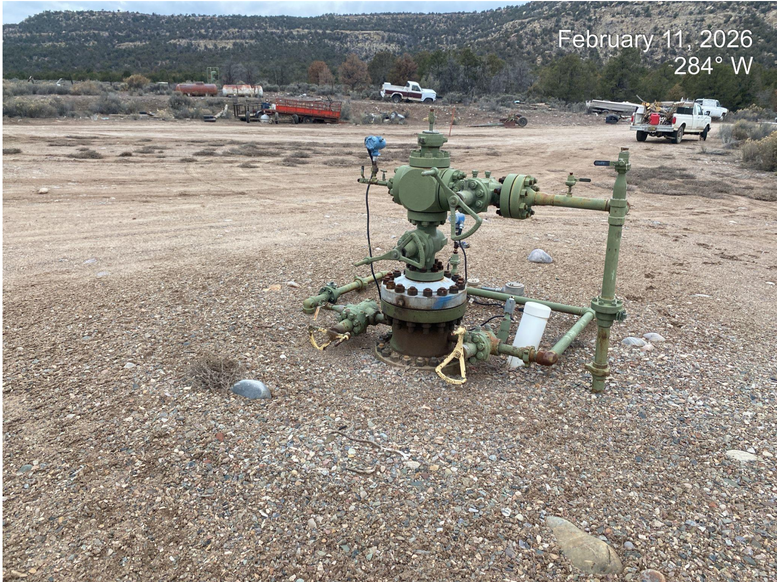
Photo 4. Wellhead assembly.
