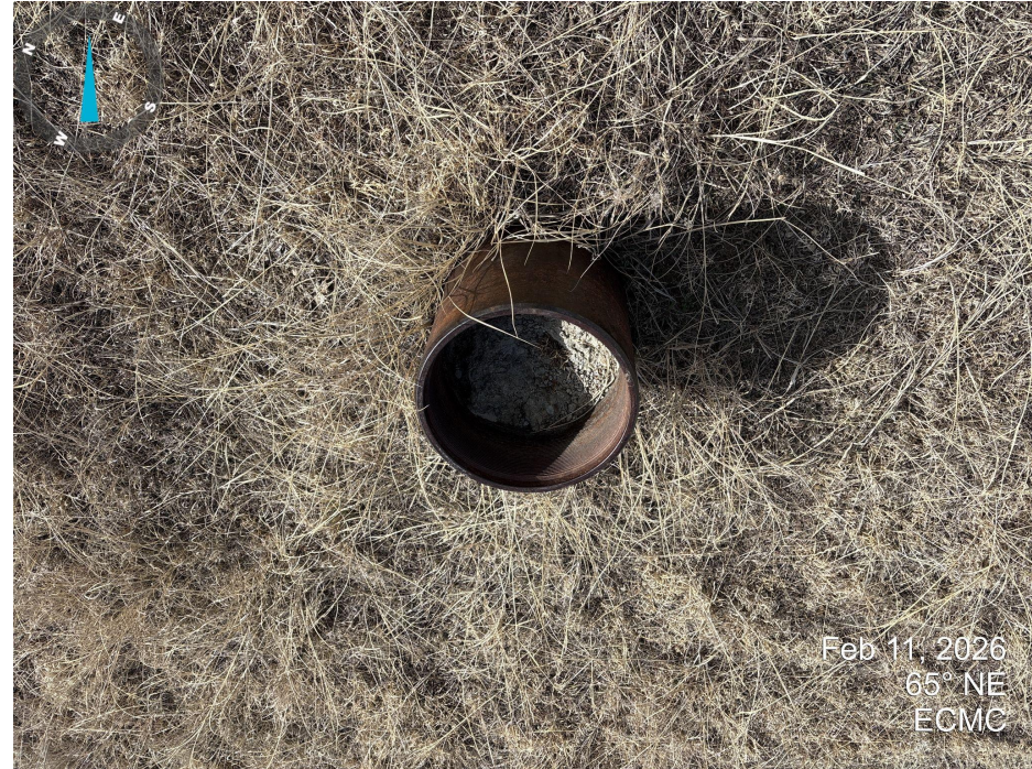
Photo 2. Picture taken on location. Surface casing is visible, filled with cement.
