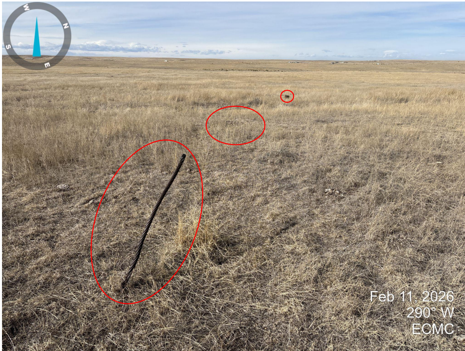
Photo 7. Picture taken approximately 50 ft to the east of the wellbore, looking west. Approximately 1.5 inch thick braided steel cable is set in ground. Also visible in this picture are ½ inch braided cable and wellbore (red circles)
