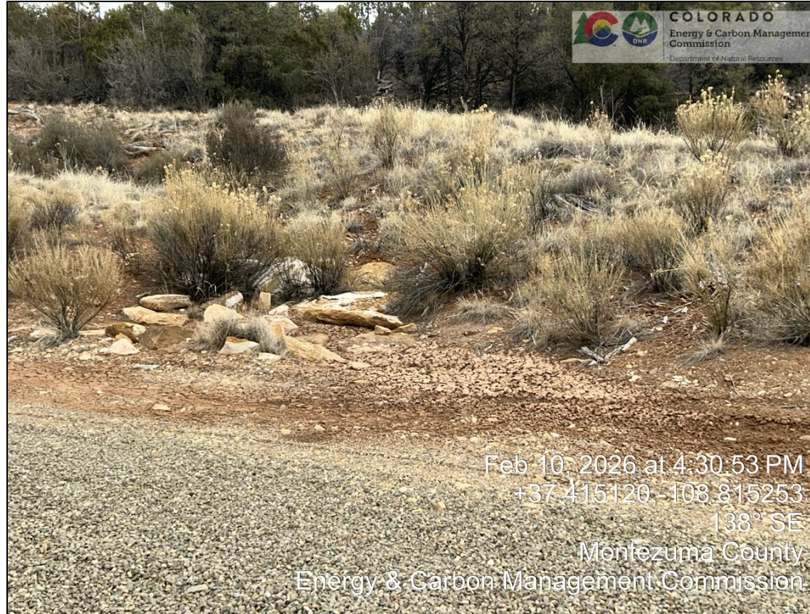
15. Location where run-on diversion ditch meets well pad.
