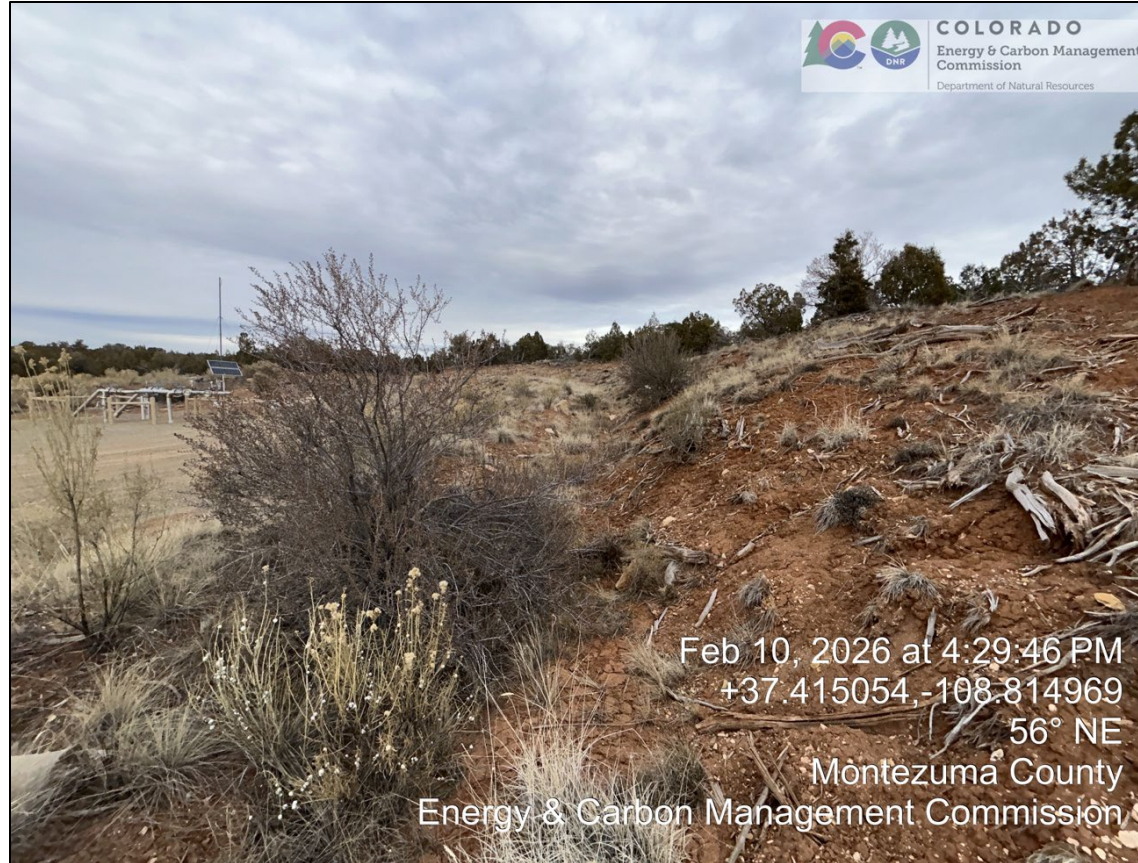
13. Run-on diversion ditch on east side of pad looking north.
